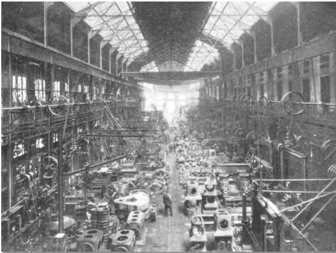
Figure 39. Interior of the main machine shop of the Westinghouse Machine Company (Walter M. McFarland, "George Westinghouse—Inventor, Organizer, and Director," The Engineering Magazine 20, no. 4, January 1901, 538).
