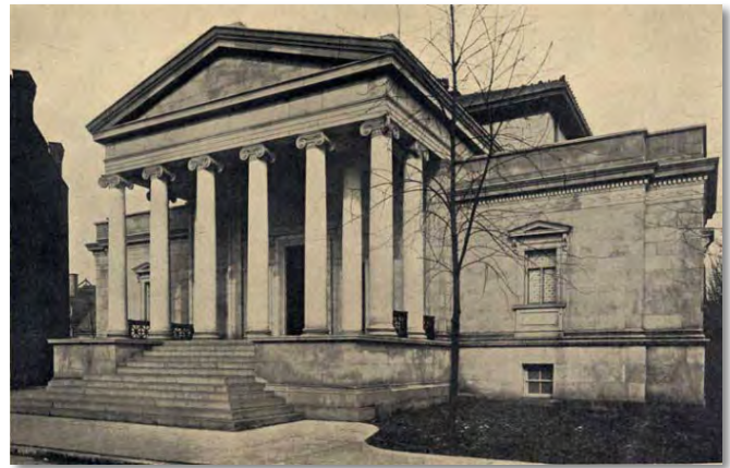
Figure 63. Former First Church of Christ, Scientist (1904) in Shadyside, designed by Chicago architect Solon Spencer Beman ( The Inland Architect and News Record , February 1907).
