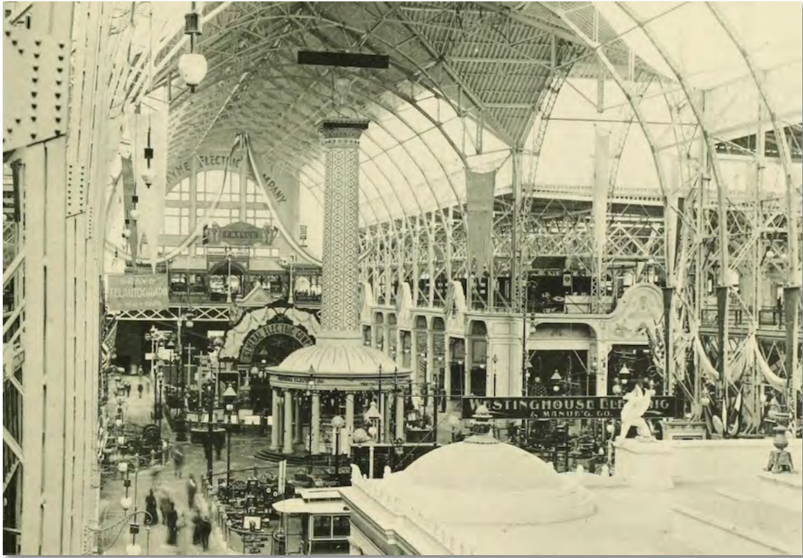
Figure 30. Interior view of the Electricity Building, showing a portion of the Westinghouse exhibits in the open center of the floor plan, which was made possible by Emil Keller's redesign ( Official Views of the World's Columbian Exposition , Plate 30).
