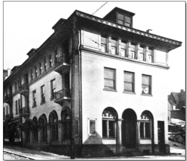
Figure 61. The First National Bank of Pitcairn (c. 1910), designed by Kiehnel and Elliott (Martin Aurand, "Prairie School Architecture in Pittsburgh").
