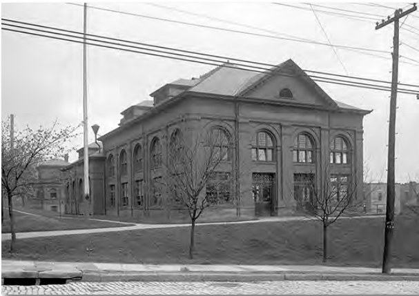
Figure 62. Herron Hill Pumping Station (1896) in North Oakland, designed by William S. Fraser, showing its front-facing pediment of Neoclassical design (Historic Pittsburgh).
