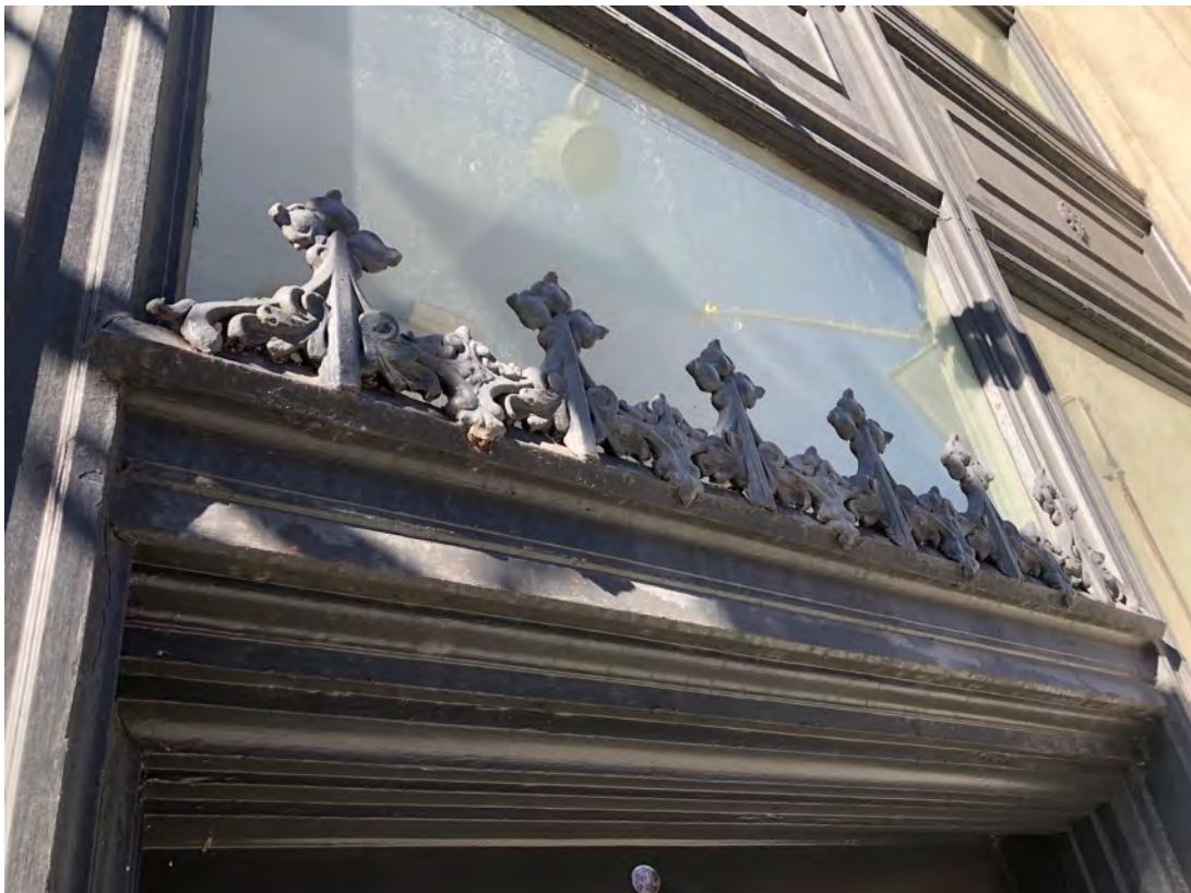
Photo 14. Front facade, looking southwest, showing detail over west entrance.
