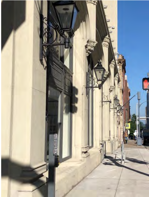
Photo 8. Front facade, sidewalk level, looking west.
