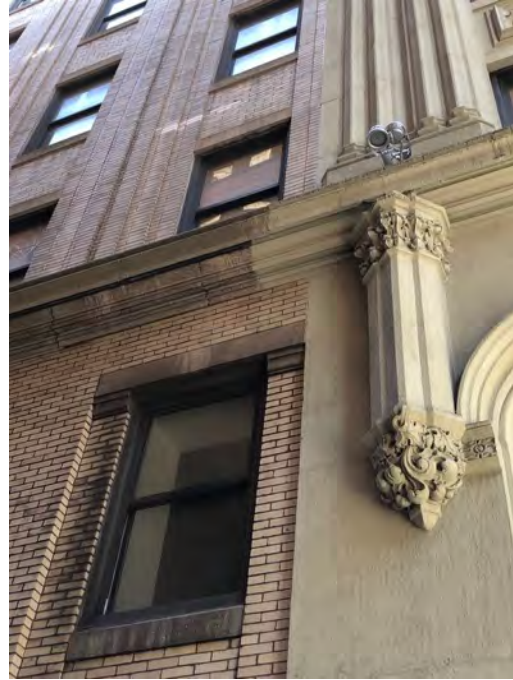
Photo 16. East facade, looking west, showing extent of painted stone.
