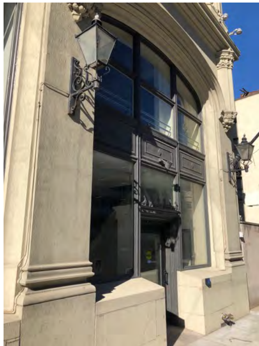
Photo 11. Front facade, looking southwest, showing west entrance.
