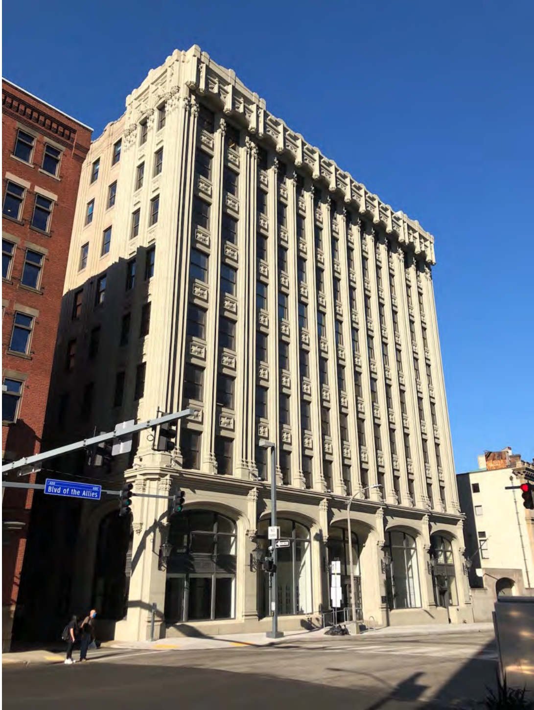
Photo 4. Front and east facades, looking southwest.
