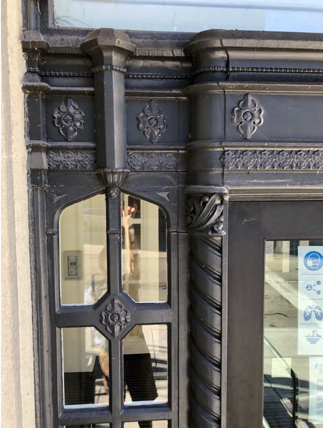
Photo 12. Front facade, looking south, showing detail at front entrance.
