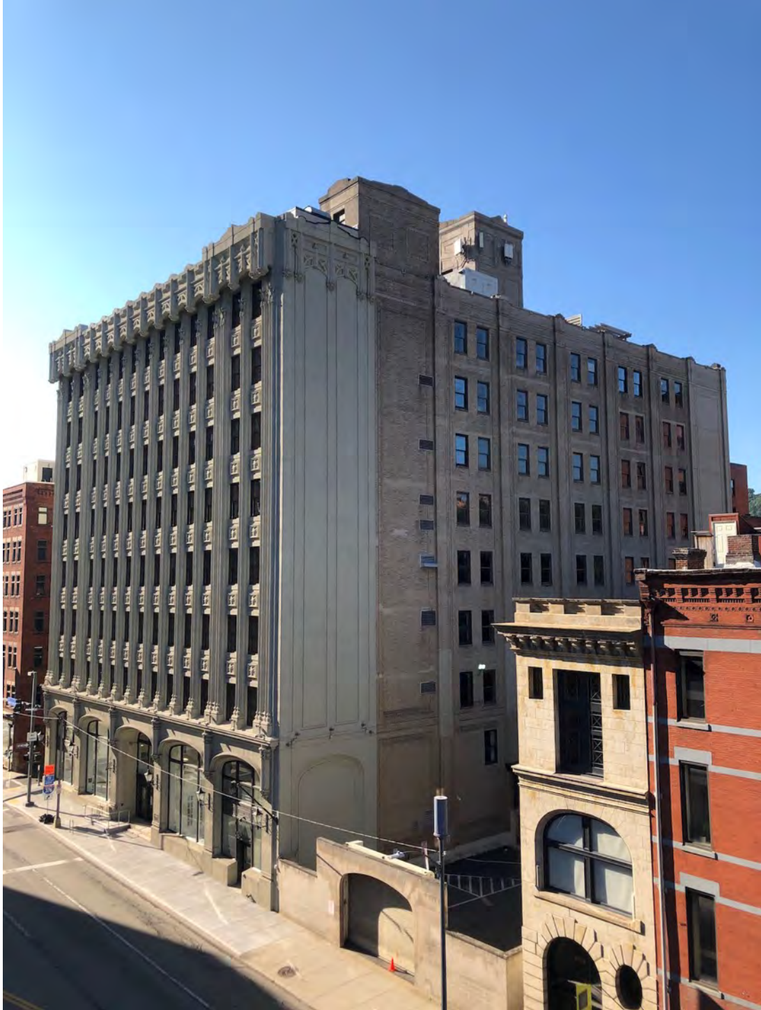
Photo 3. Front and west facades, looking southeast.
