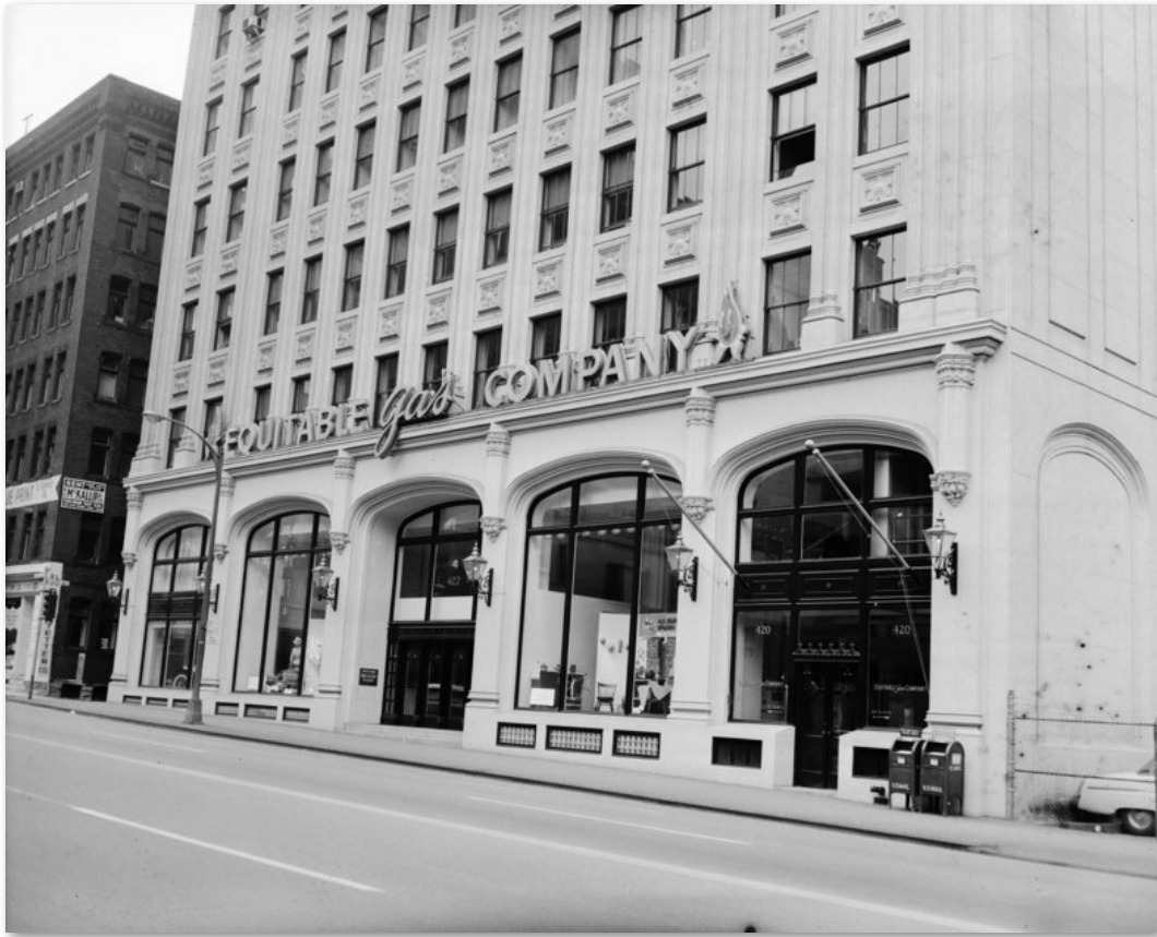
Figure 44. Front facade of Equitable Gas during their diamond-anniversary year, showing how the company utilized the front showcase windows for displays and merchandising (Teenie Harris, Carnegie Museum of Art, August 1963).
