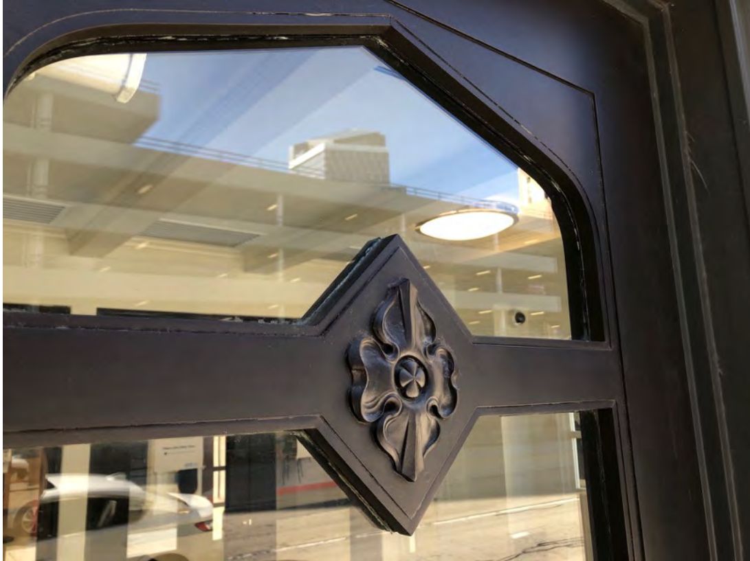
Photo 13. Front facade, looking southwest, showing detail on front door.
