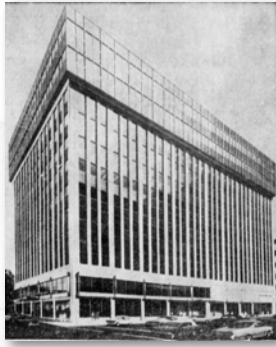
Figure 48 (inset, at left). Mid-1960s renovations added two floors to the McCann Building and covered all vestiges of its Commercial Gothic past (Pittsburgh Press, 14 April 1968).
