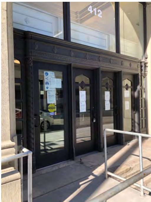
Photo 10. Front facade, looking southwest, showing main entrance.
