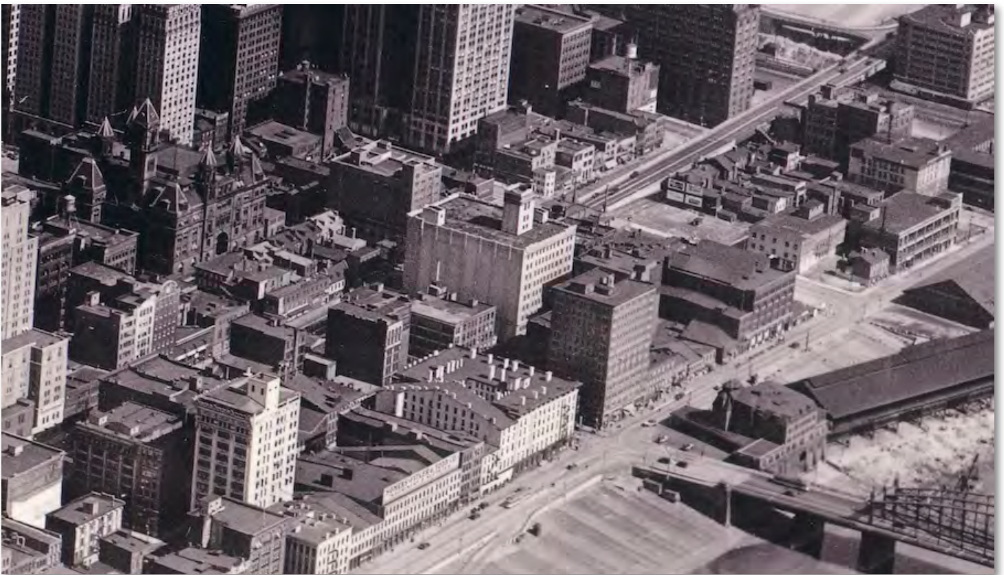
Figure 14. Another early view of the new Gilmore Building (center), showing the absence of windows on the west facade (Dallin Aerial Survey Collection, Hagley Museum and Library, 9 September 1932).
