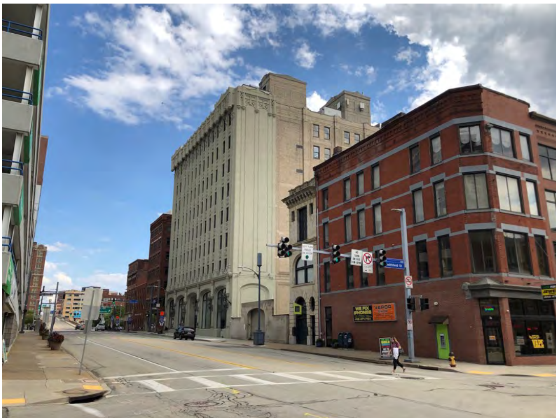
Photo 2. Streetscape; Boulevard of the Allies, looking east from Smithfield Street, showing 412 Boulevard of the Allies in the middle of the block on the right.
