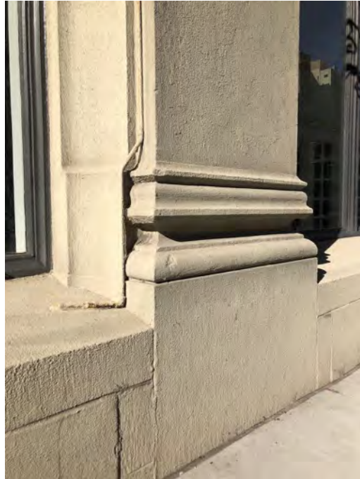
Photo 9. Front facade, looking southwest, showing base of pilaster and painted surfaces.
