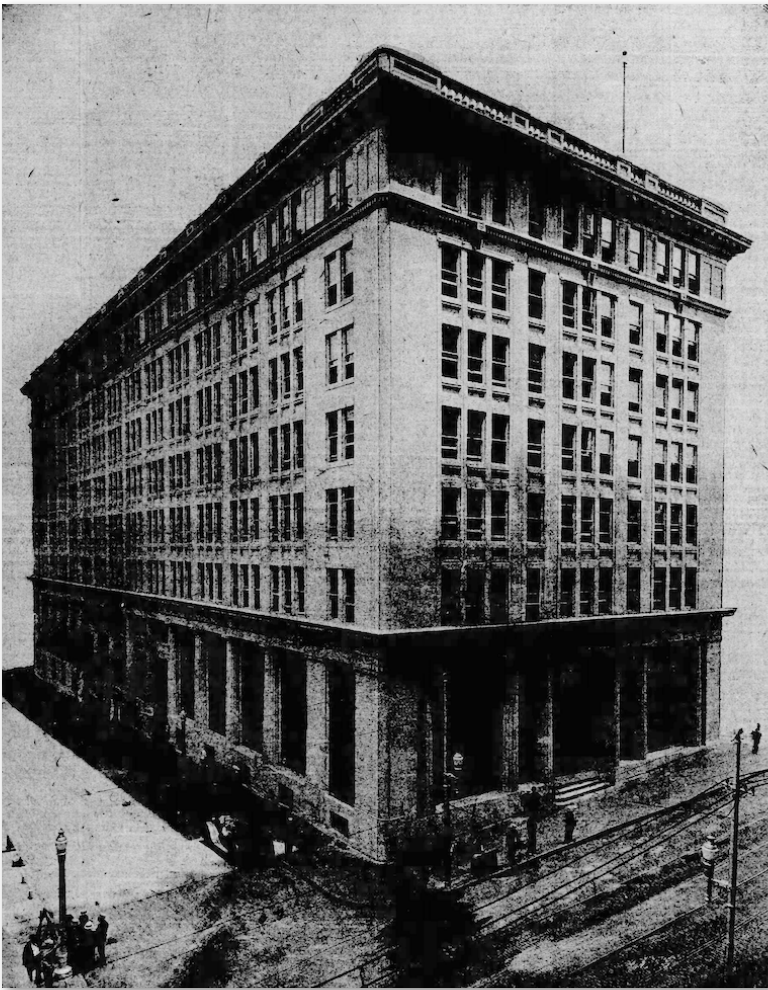
Figure 61. Joseph Kuntz designed to expansion of the Philadelphia Company headquarters (1925). Twenty-five years later, Equitable Gas would spin off and move into what was then 420 Boulevard of the Allies. Today, this is the Hotel Monaco ( Pittsburgh Post-Gazette , 25 June 1925)
