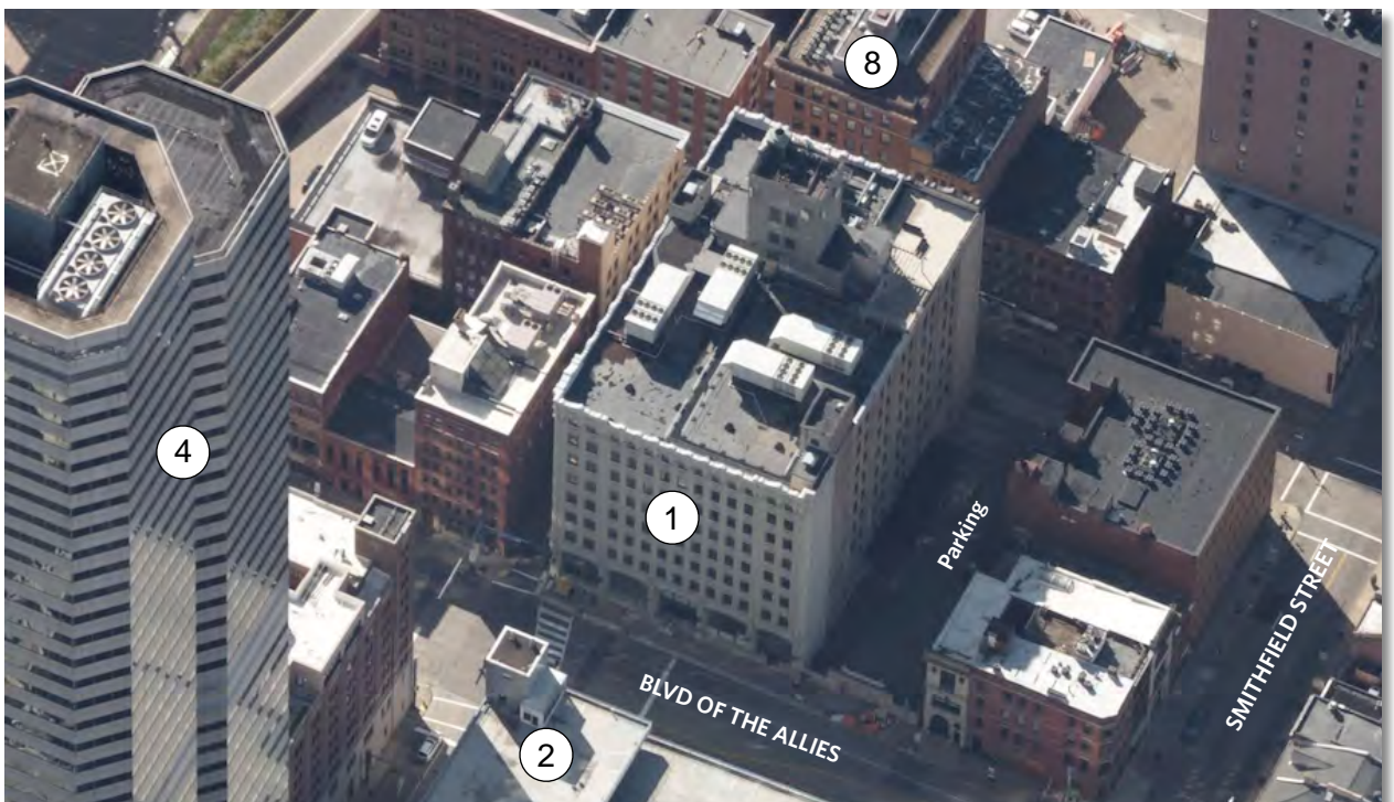
Figure 3. Vicinity plan. Birdseye view, looking south, showing roof of 412 Boulevard of the Allies (Bing Maps).
