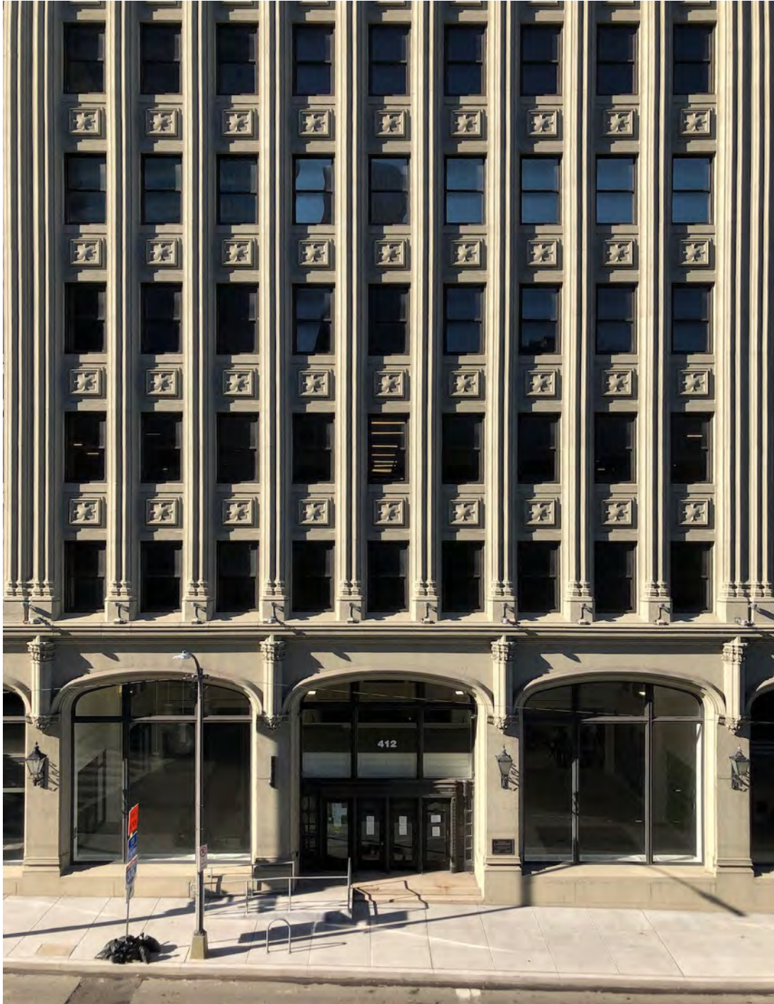
Photo 5. Front facade, center three bays, looking south.
