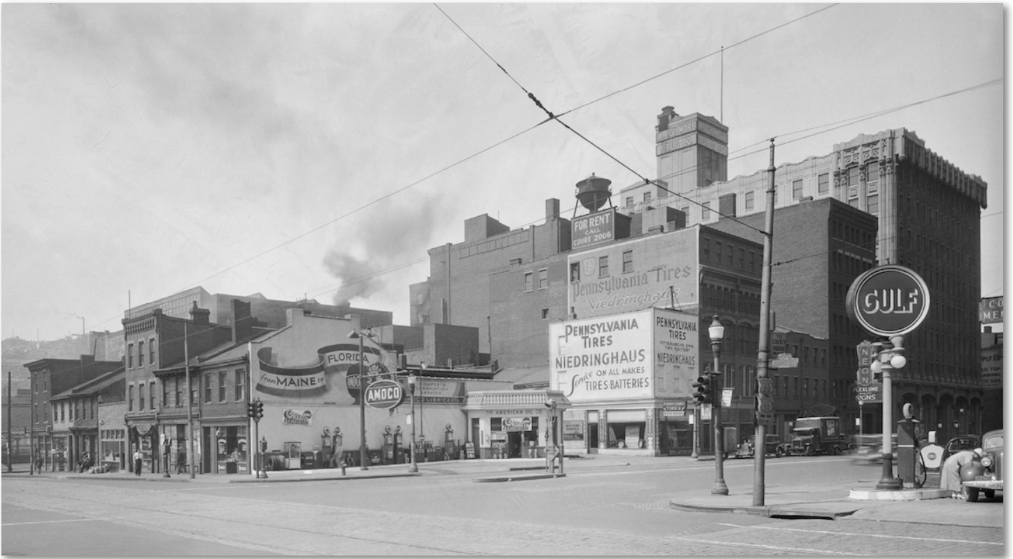
Figure 13. A view of the recently-completed Gilmore Drug Company Building (upper right), looking southwest from the intersection of the Boulevard of the Allies and Grant Street. Wrapping the elevator penthouse are signs for “W.J. Gilmore Drug Co.” (Pittsburgh City Photographer Collection, Historic Pittsburgh, 1935).
