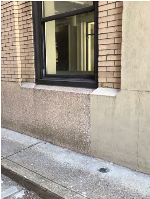
Photo 17. East facade, looking west, showing extent of painted stone.
