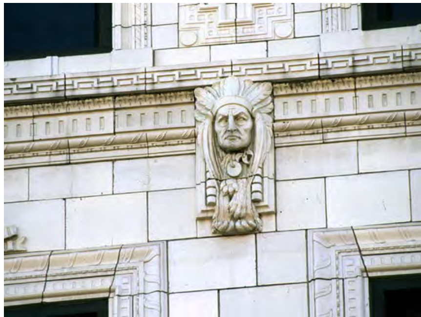
Figure 57. The Maul Building, showing a terra cotta detail (Pittsburgh History & Landmarks Foundation).
