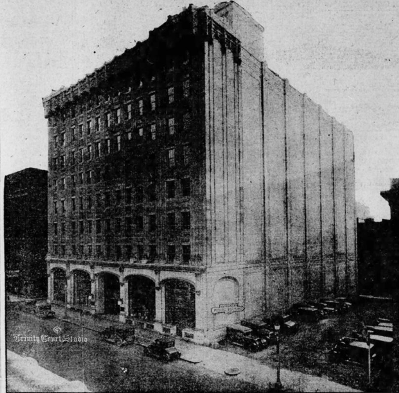
The new home of the W. J. Gilmore Drug Co. is in the United States. It has eight stories and a mezzanine located at Second ave. Cherry way and First ave. The exterior is of stone and gray vitrified construction of the building. Joseph F. Kuntz was the architect.
