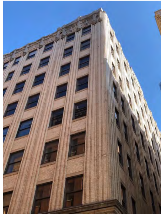
Photo 20. Rear and east facades, looking northwest, showing similar brickwork.
