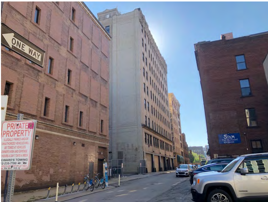
Photo 21. Rear facade, looking east.
