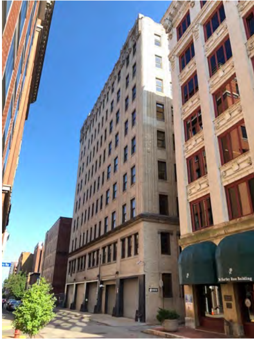
Photo 19. Rear facade, looking west.
