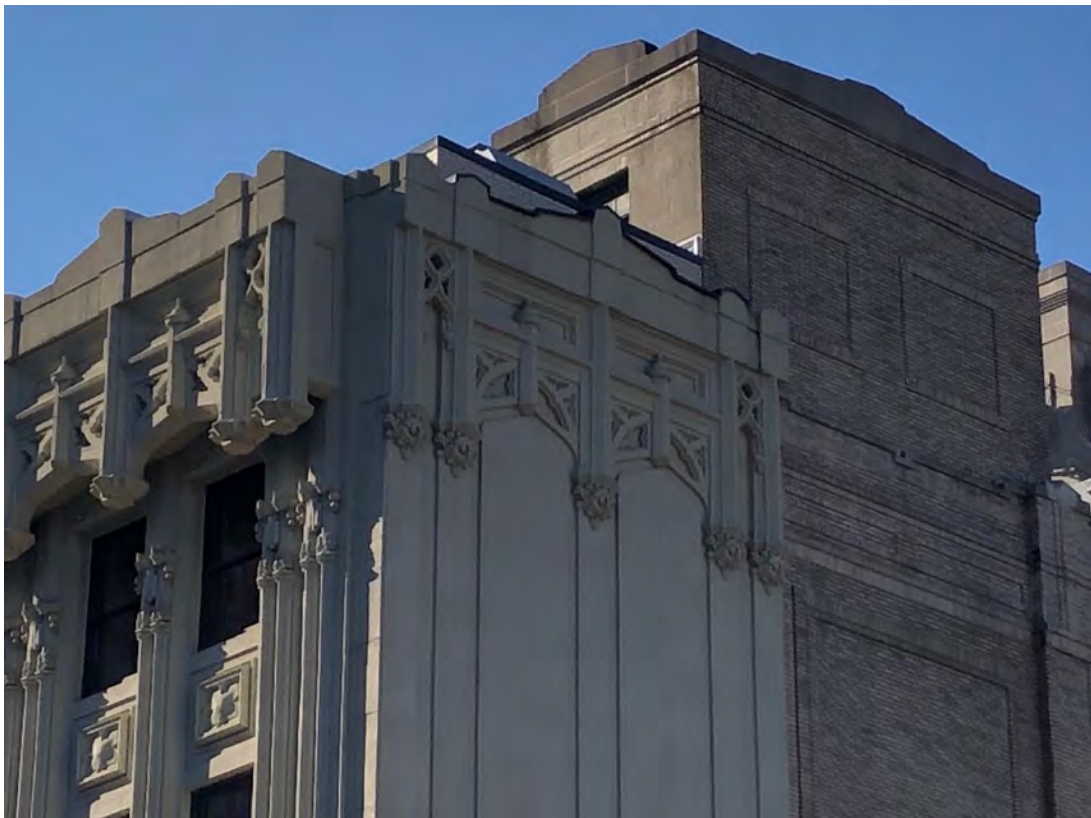
Photo 7. Detail, cornice, northwest corner of building, looking southeast.
