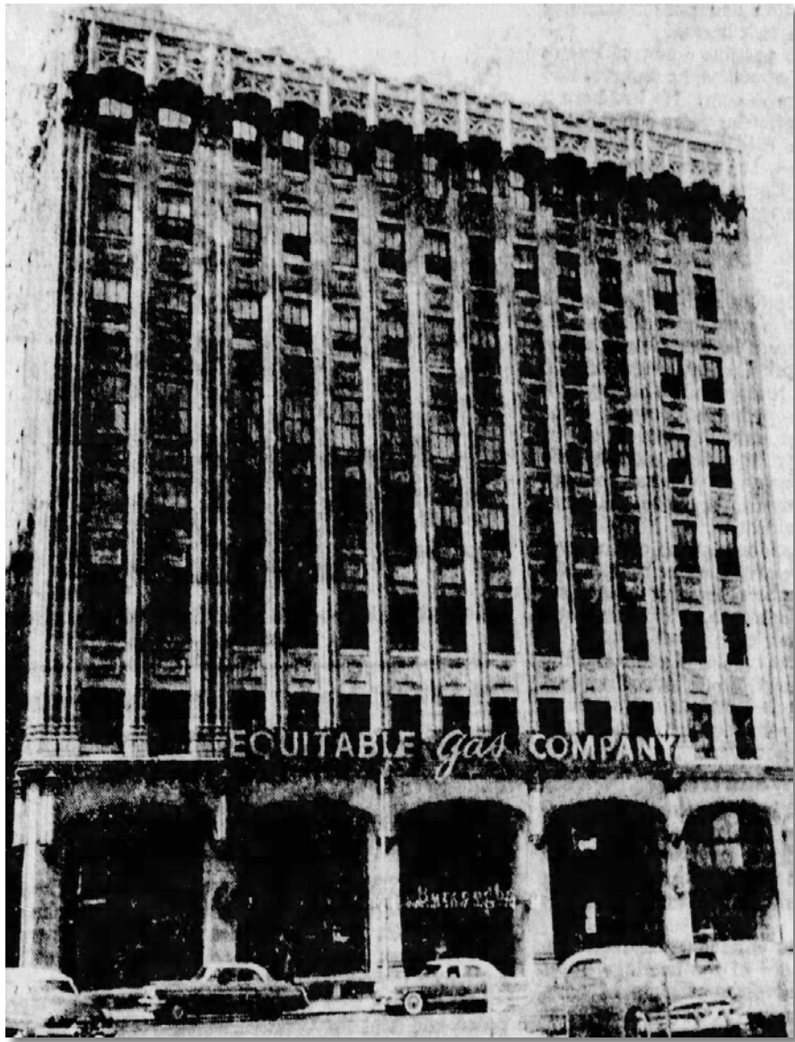
Figure 15. Front facade of the new Equitable Gas Company headquarters, showing the original three-over-three , metal, double-hung sash windows and the company's new sign ( Pittsburgh Sun-Telegraph , 23 June 1953).
