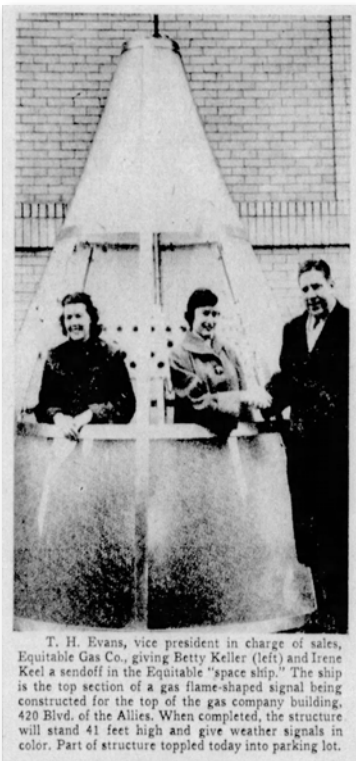
Figure 37. Top section of the Weather Flame just before installation ( Pittsburgh Sun-Telegraph , 15 December 1955)
