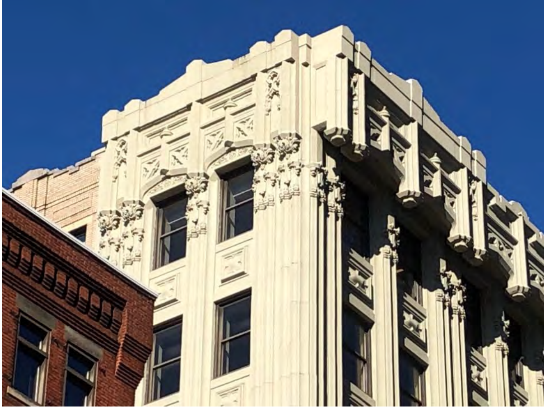
Photo 6. Detail, cornice, northeast corner of building, looking southwest.
