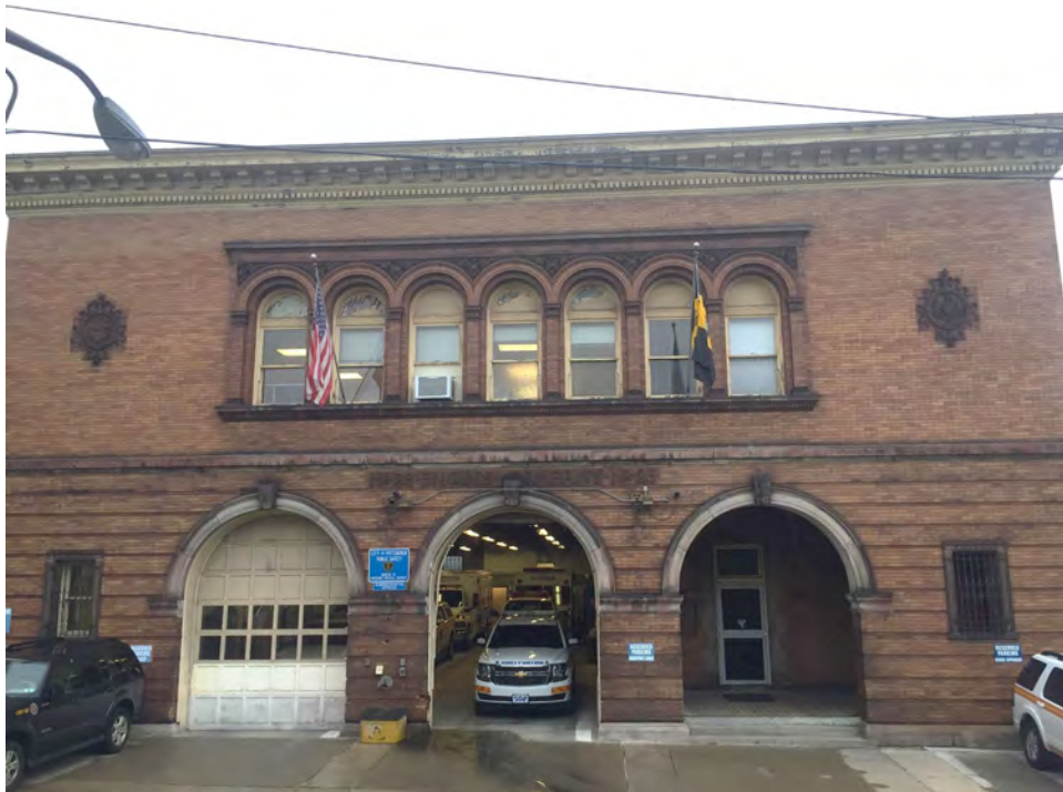
Photograph 2. Pittsburgh EMS Station, Filbert Street Facade, Facing Southwest. Source: Calvin A Yoder.
