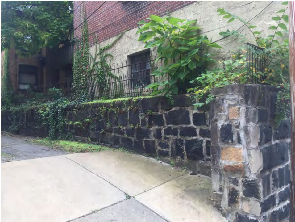
Photograph 20. Pittsburgh EMS Station, Southern Fence, Facing Southeast. Source: Calvin A Yoder.
