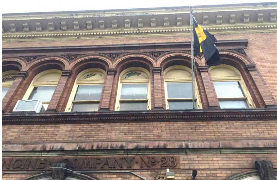
Photograph 6. Pittsburgh EMS Station, Filbert Street Facade, Second Story Arcading, Facing Southwest. Source: Calvin A Yoder.
