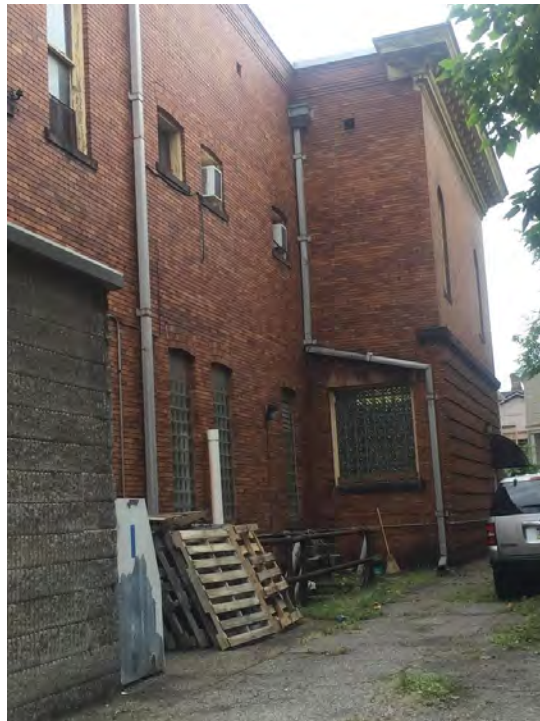
Photograph 16. Pittsburgh EMS Station, Southern Facade, Facing Northeast. Source: Calvin A Yoder.
