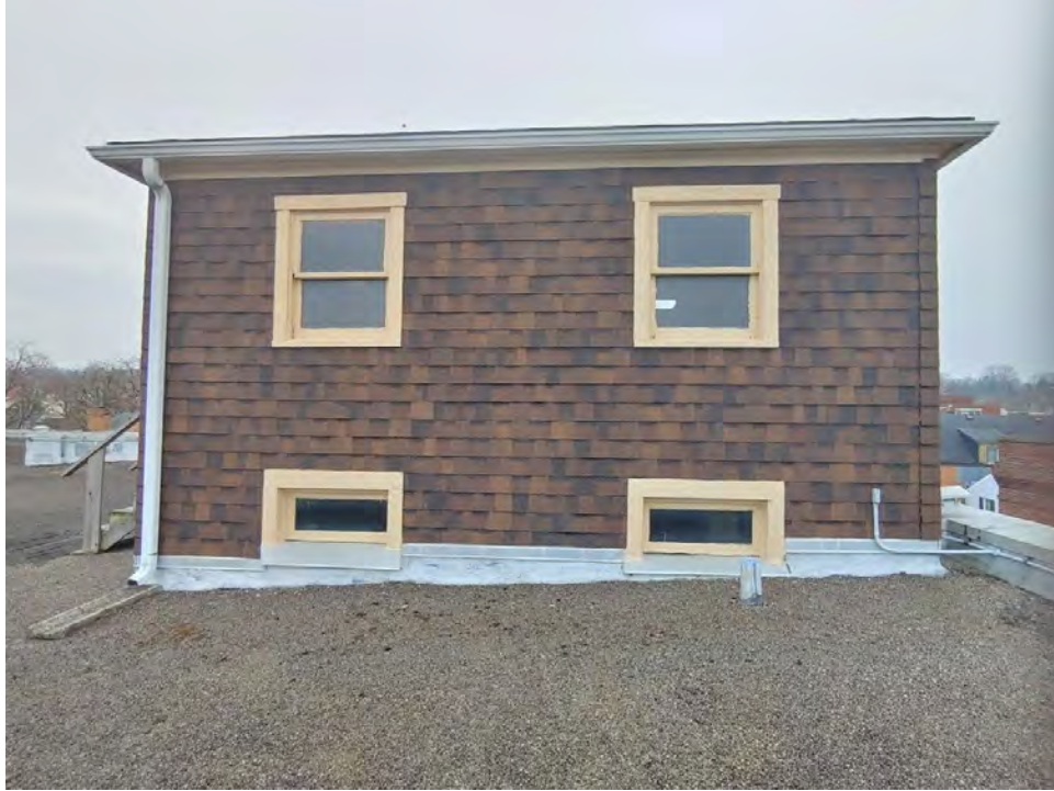
Photograph 27. Pittsburgh EMS Station, Hose Tower, Facing Southeast. Source: Dana Cress.
