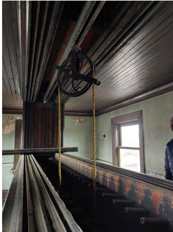
Photograph 28. Pittsburgh EMS Station, Hose Tower, Interior. Source: Dana Cress.
