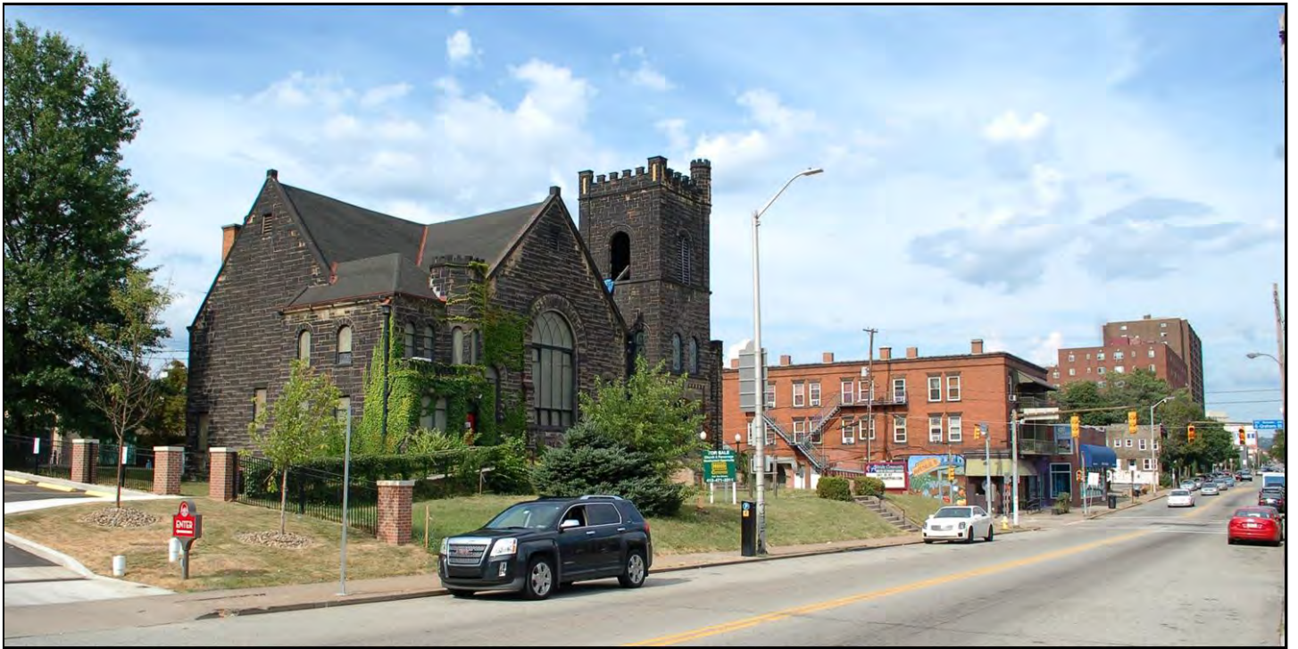
Photo 5: Albright United Methodist Church in context looking east on Centre Avenue, August 2015. Source: Justin Greenawalt
