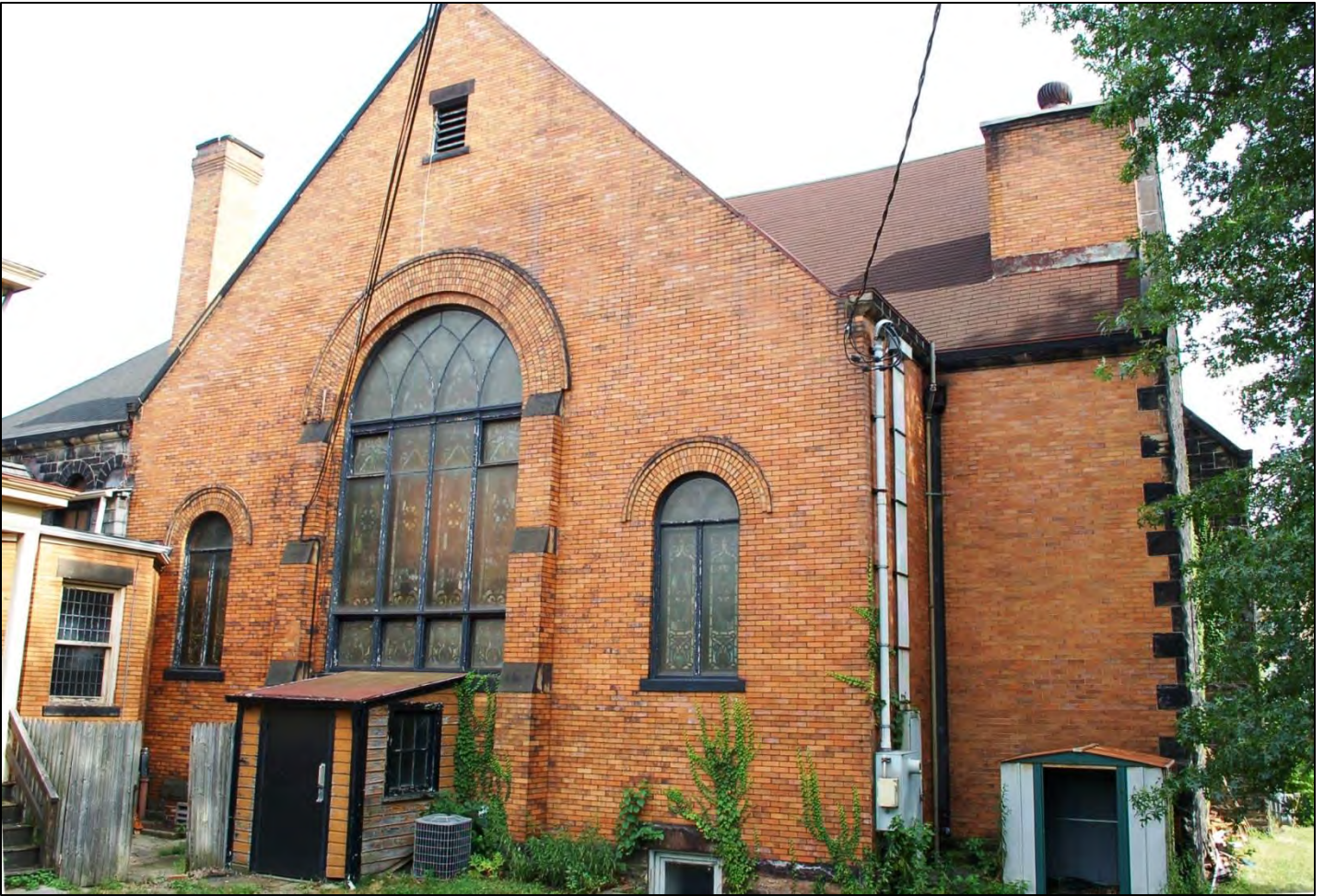
Photo 9: Albright United Methodist Church, northern facade, August 2015. Source: Justin Greenawalt
