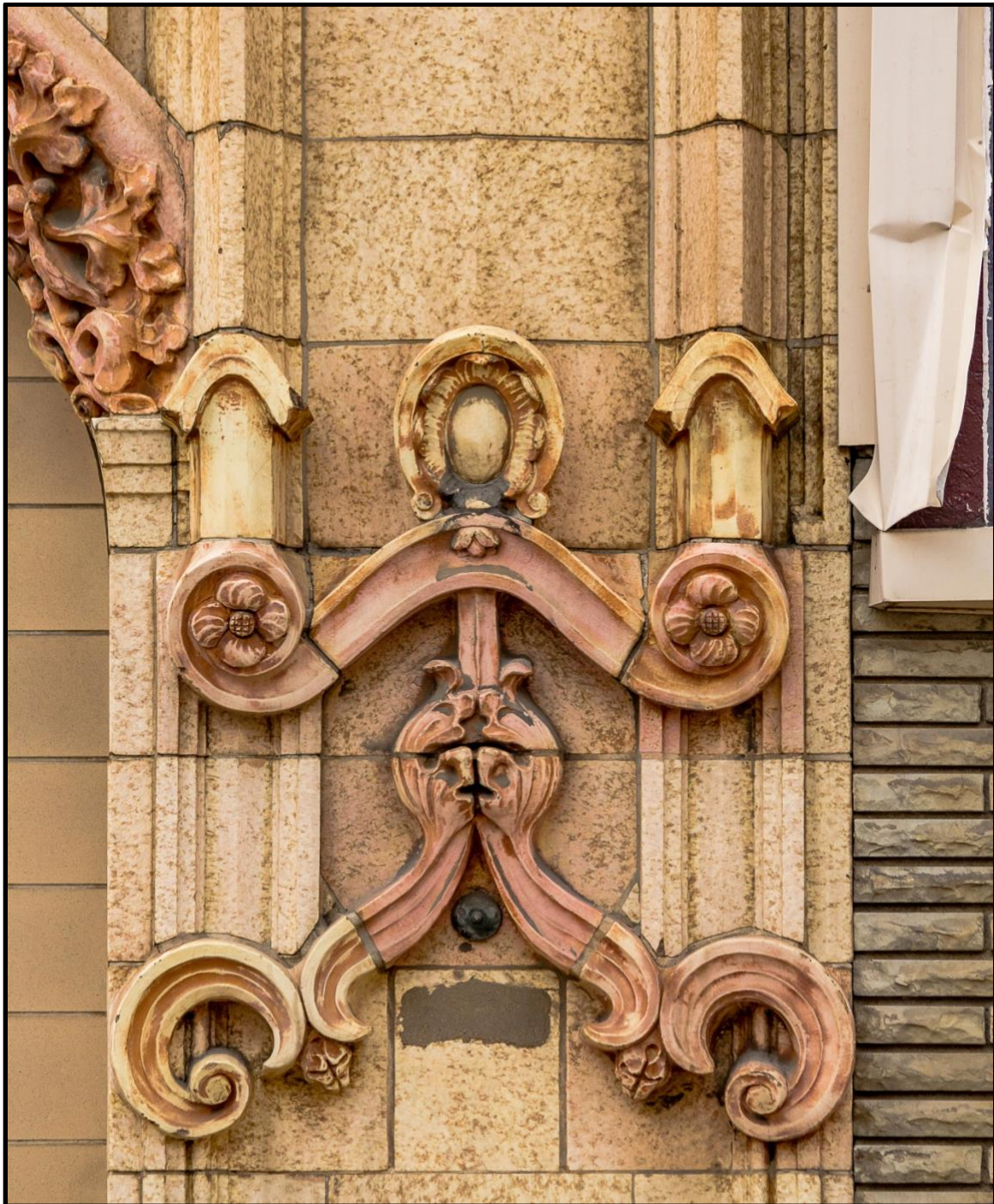
Photo 6: Light fixture terra cotta scrollwork. Source: Amy Fisher
