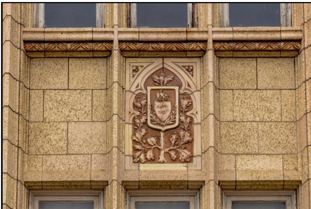
Photo 8: Spandrel with arch and escutcheon. Source: Amy Fisher
