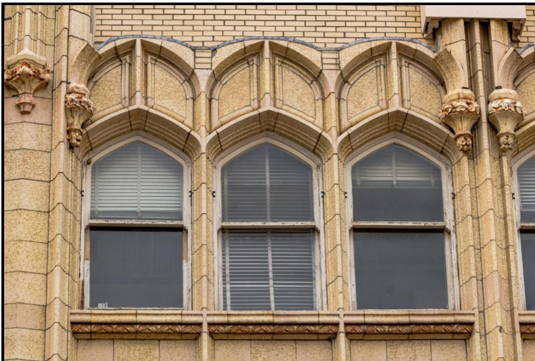
Photo 10: Blind parapet arcade. Source: Amy Fisher
