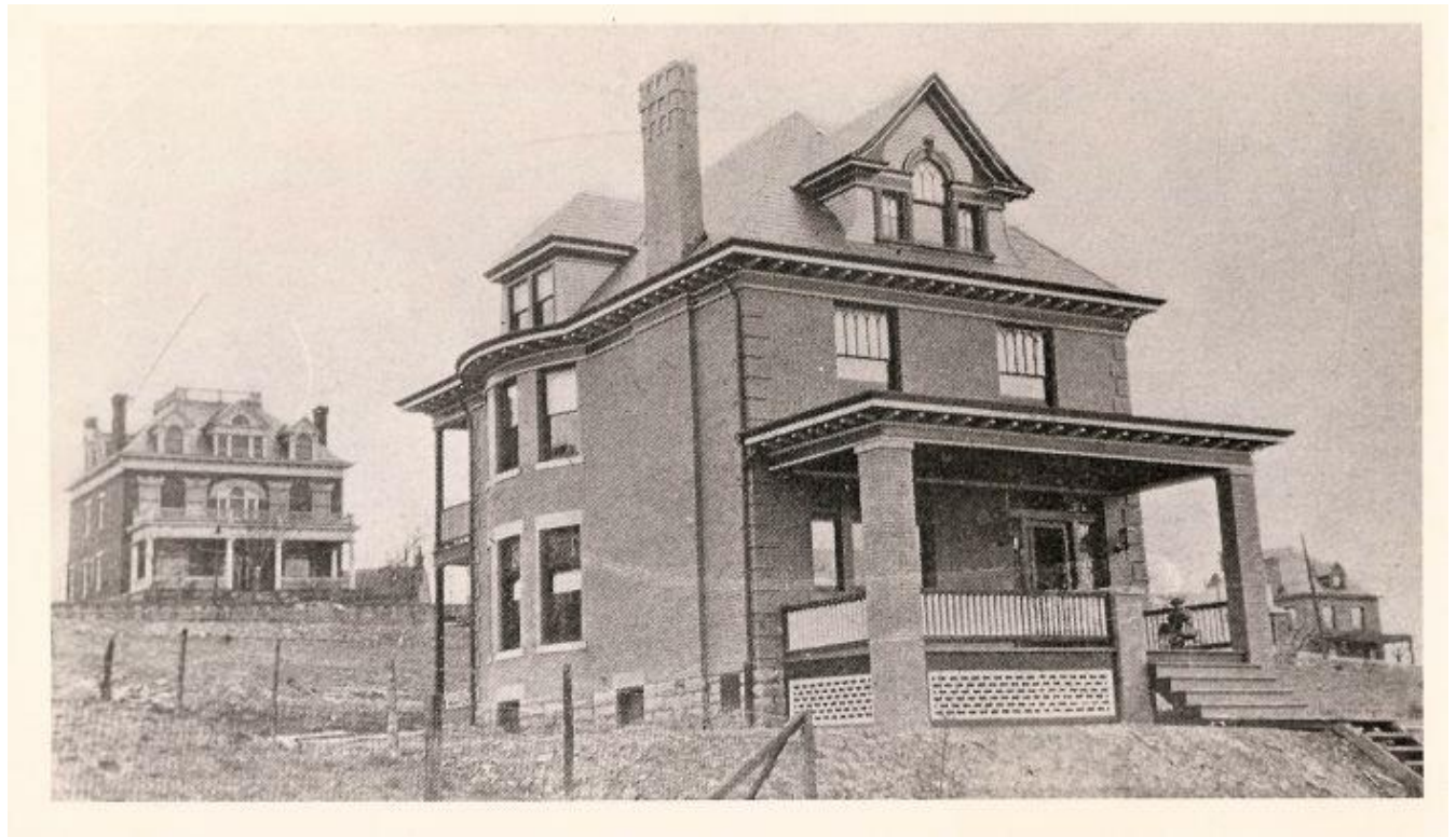
Figure 2: Historical photograph of the Sankey Mansion (background).
