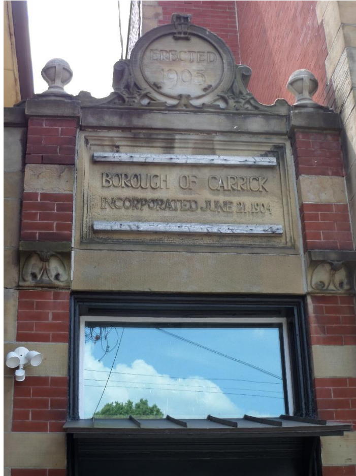
Photo. 7. Borough of Carrick Dedication Stone, Carrick Municipal Building Stone Medallion, Former Carrick Municipal Building, Brownsville Road Façade, June 18, 2018. Source: Antonio Parente.
