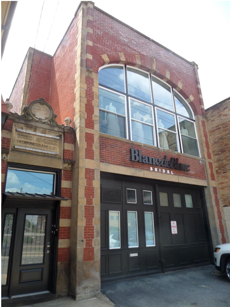
Photo. 3. Former Carrick Municipal Building, Brownsville Road Façade , June 18, 2018. Source: Antonio Parente.
