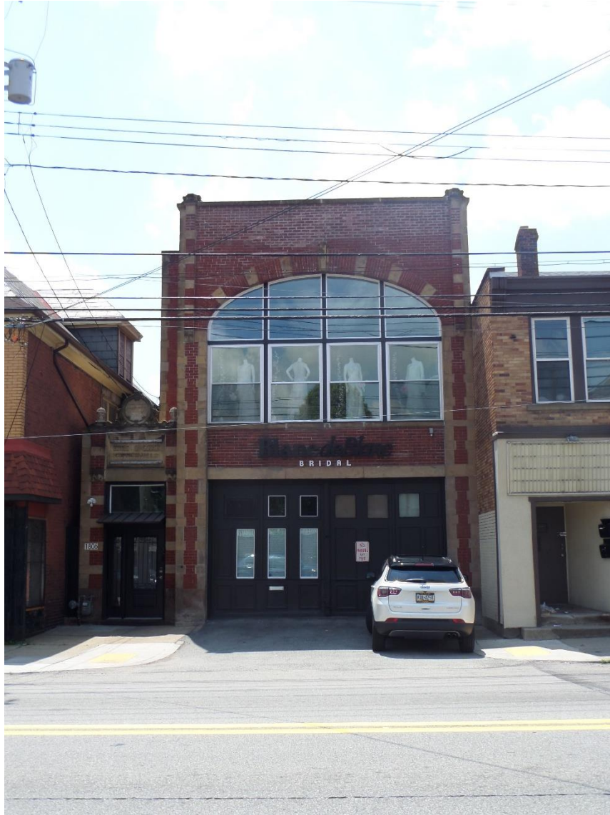
Photo. 1. Former Carrick Municipal Building, Brownsville Road Façade , June 18, 2018. Source: Antonio Parente.
