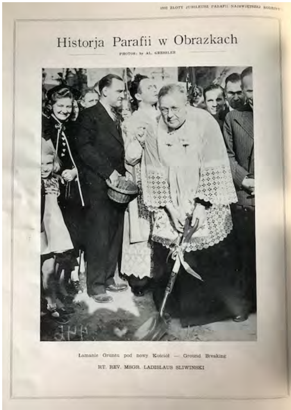
Fig. 5. Ground Breaking, The Holy Family Church Golden Jubilee , 1952.
