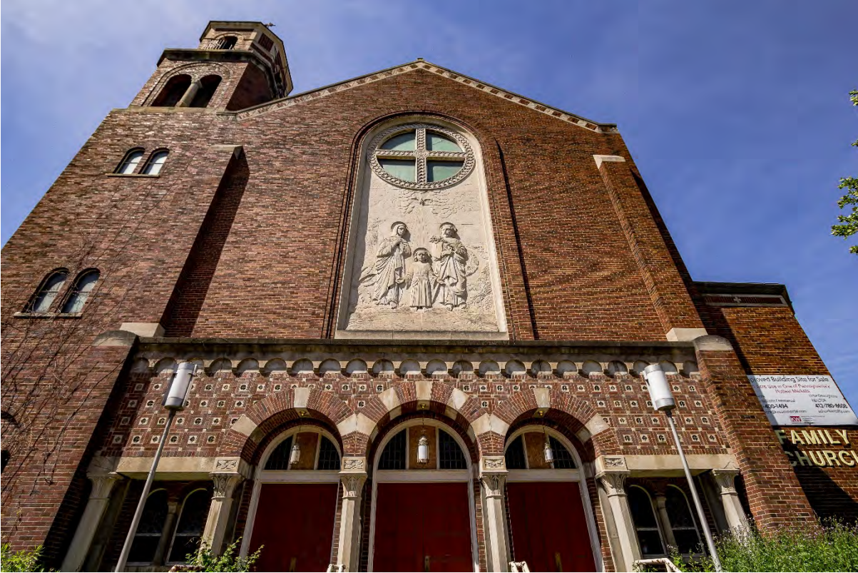
Photo. 1. Former Holy Family Church, 44 th St. (Primary) Façade, June, 2018. Source: Preservation Pittsburgh.
