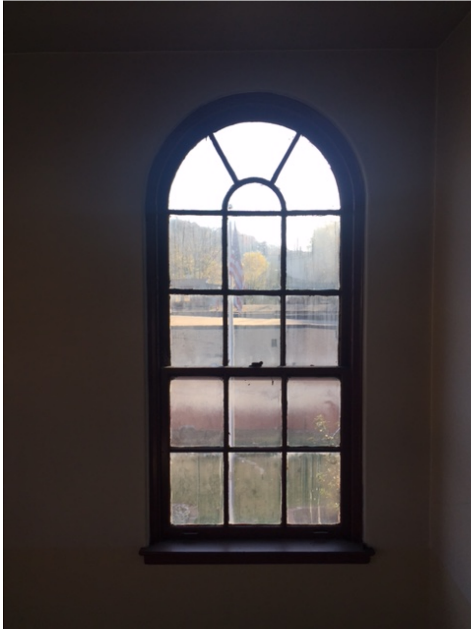
Photo. 12. Former Overbrook Municipal Building, Stairwell Window , March 2, 2017. Source: Matthew W.C. Falcone.
