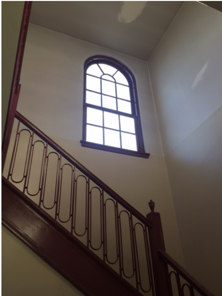
Photo. 11. Former Overbrook Municipal Building, Interior Stairwell , March 2, 2017. Source: Matthew W.C. Falcone.
