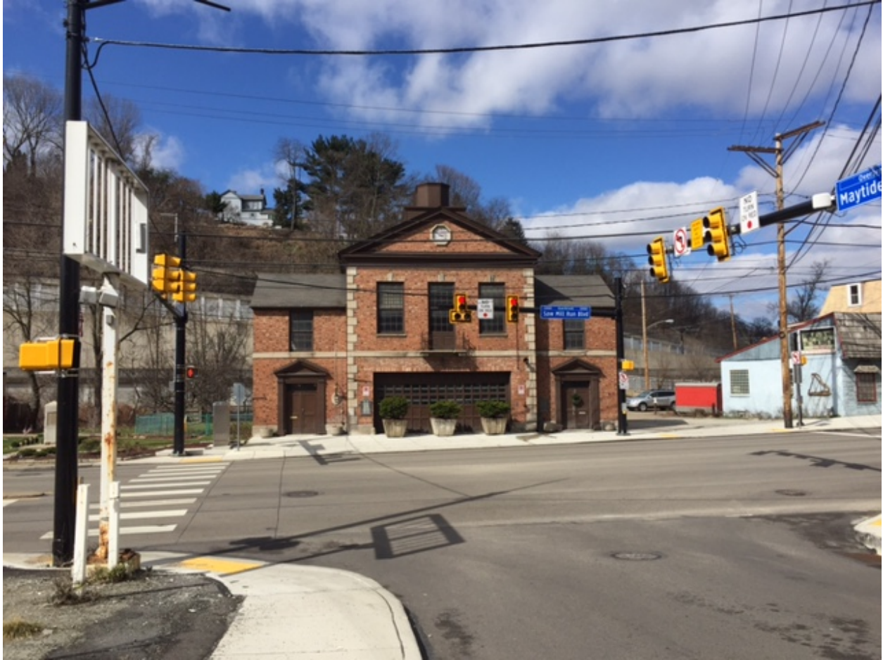
Photo. 9. Former Overbrook Municipal Building, Saw Mill Run Boulevard Façade , March 2, 2017. Source: Matthew W.C. Falcone.
