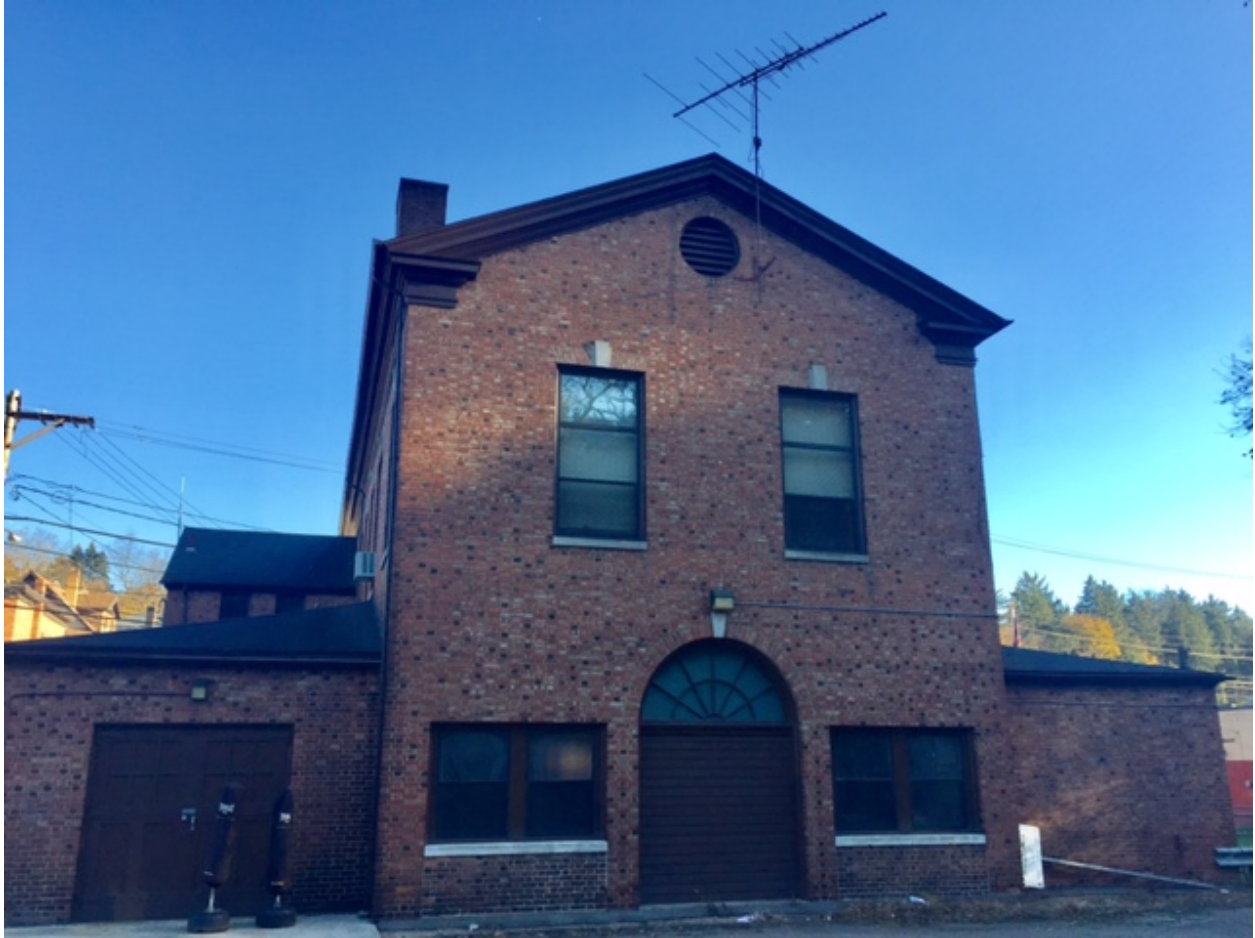
Photo. 7. Rear Façade, Former Overbrook Municipal Building, Saw Mill Run Boulevard Façade, March 2, 2017. Source: Matthew W.C. Falcone.
