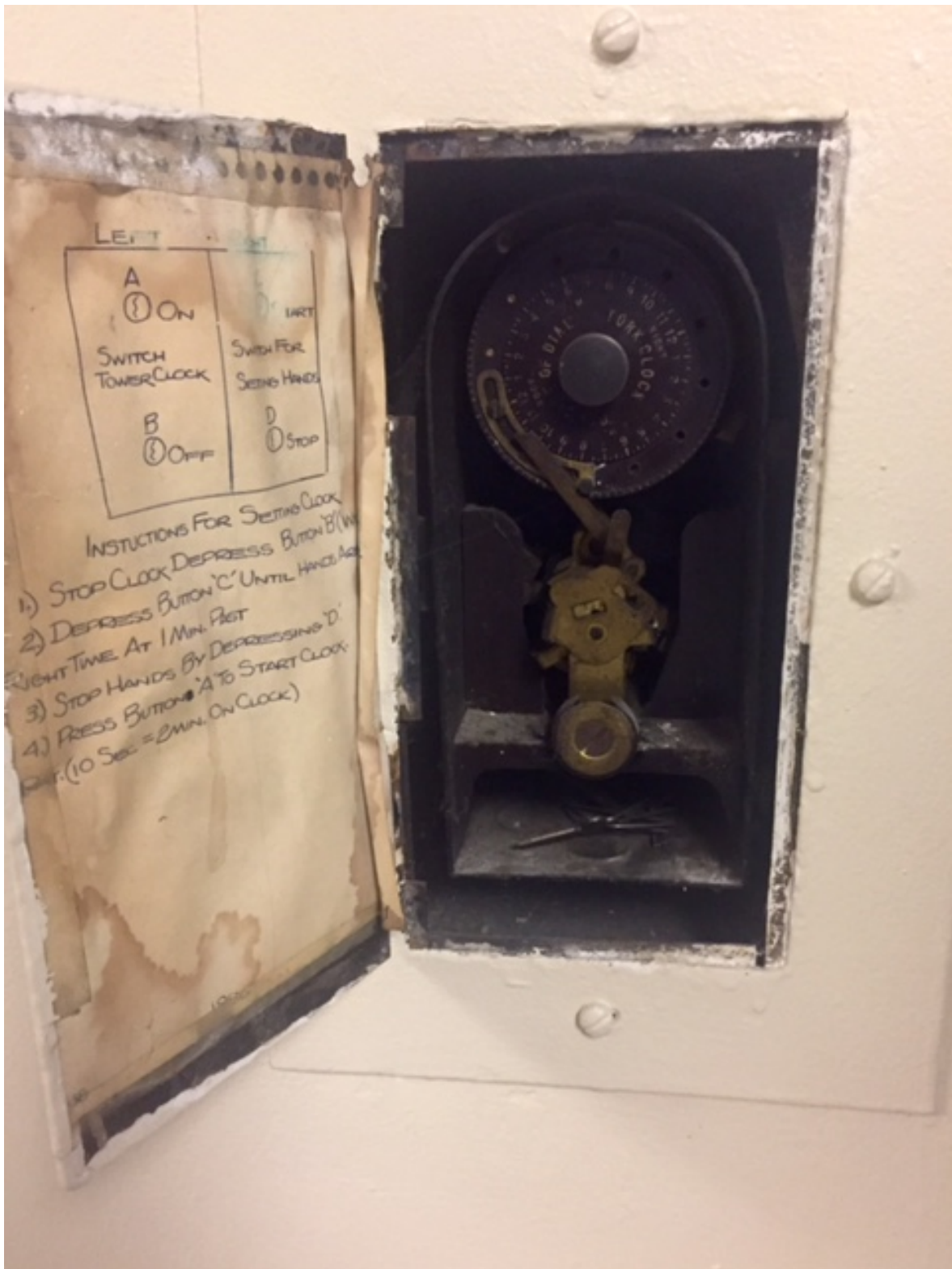
Photo 10. Former Overbrook Municipal Building, Clock Controls, March 2, 2017. Source: Matthew W.C. Falcone.
