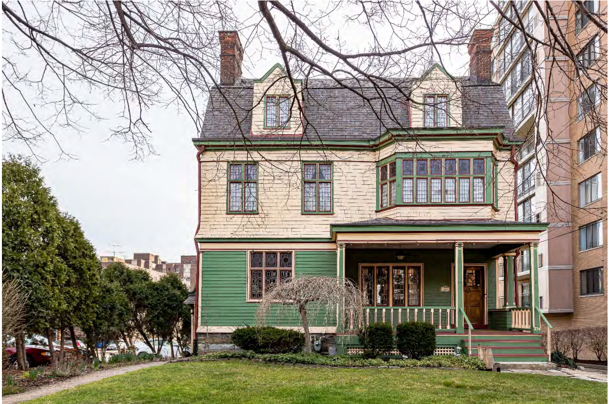
Photo. 2. Gallagher-Kieffer House, Southwest (Front) Façade , March 2020. Source: Matthew W.C. Falcone.
