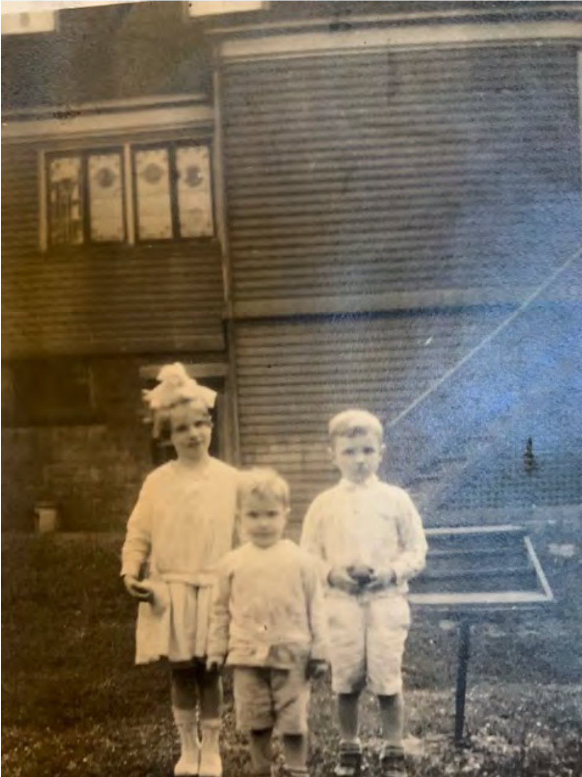
234 N. Dithridge Street, Detail of the Rear of the House. Private Collection of Kathy Gallagher. In contrast to the previous image, the dining room windows have been replaced with what appears to be leaded-and-stained glass. The glazing program in the dining room today is leaded grisaille glass, suggesting the windows featured in this photograph were replaced and the stained-glass medallions appear to reflect the same subjects as those currently in the entryway (lighthouse, garden, ship, castle).
