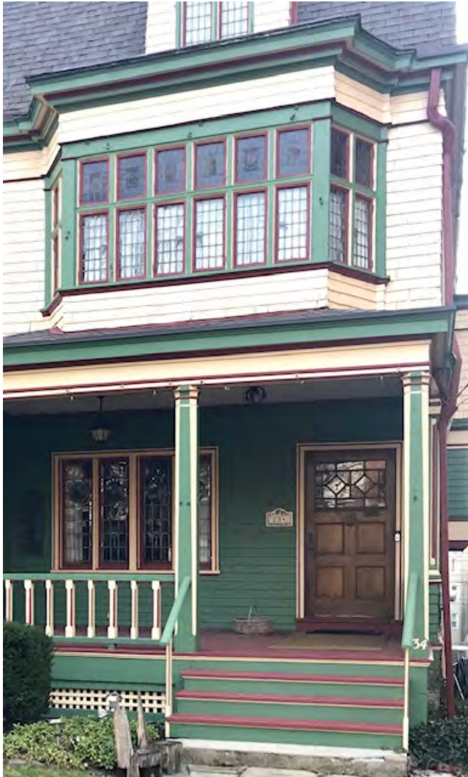
Photo. 10. Gallagher-Kieffer House, Library Windows (Exterior) , March 2020. Source: Matthew W.C. Falcone.
