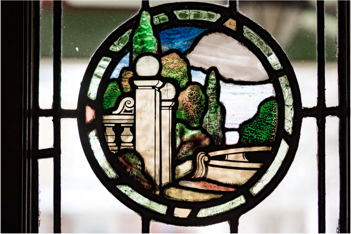
Photo. 5. Gallagher-Kieffer House, "Garden," Foyer Window Detail, March 2020. Source: Amy Fisher.
