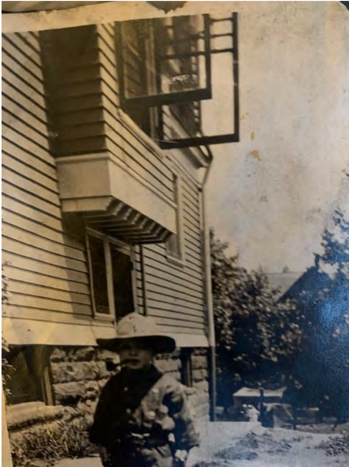
234 N. Dithridge Street, Side of the House. Private Collection of Kathy Gallagher. Note the clear-paned open windows on the second floor (the space corresponds to the main stair landing) provide insight to the fenestration prior to the current leaded-and-stained glass that occupy the opening.
