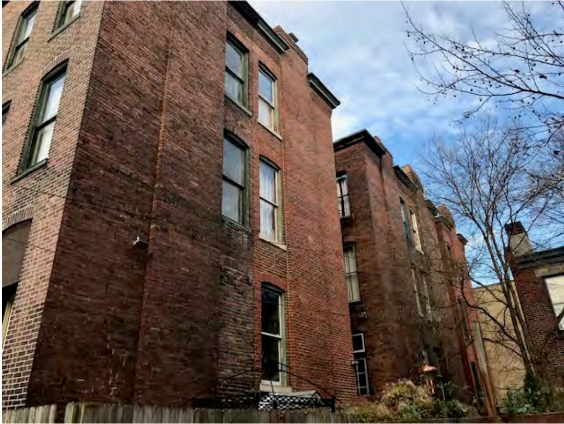
Photo. 6. 417 Lockhart Street, Rear of structure (2 nd from left) from Moravian Way. December, 2019. Source: Matthew W.C. Falcone.
