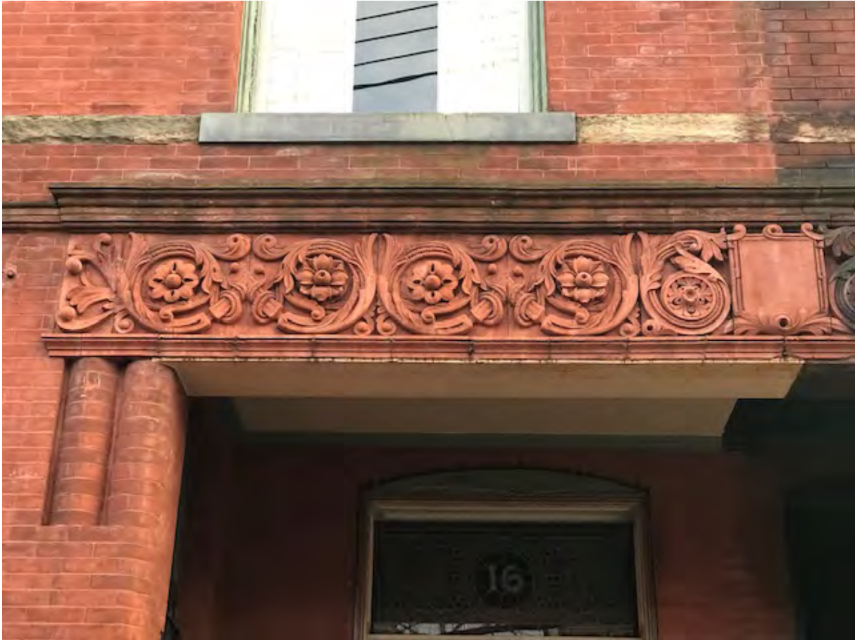
Photo. 3. 417 Lockhart Street, Primary Façade, scroll engraving & transom stained glass with original house numbering. December, 2019. Source: Matthew W.C. Falcone.
