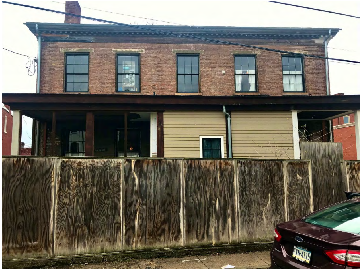
Photo 9. Echo , Rear Elevation, January 10, 2020. Source: Preservation Pittsburgh.
