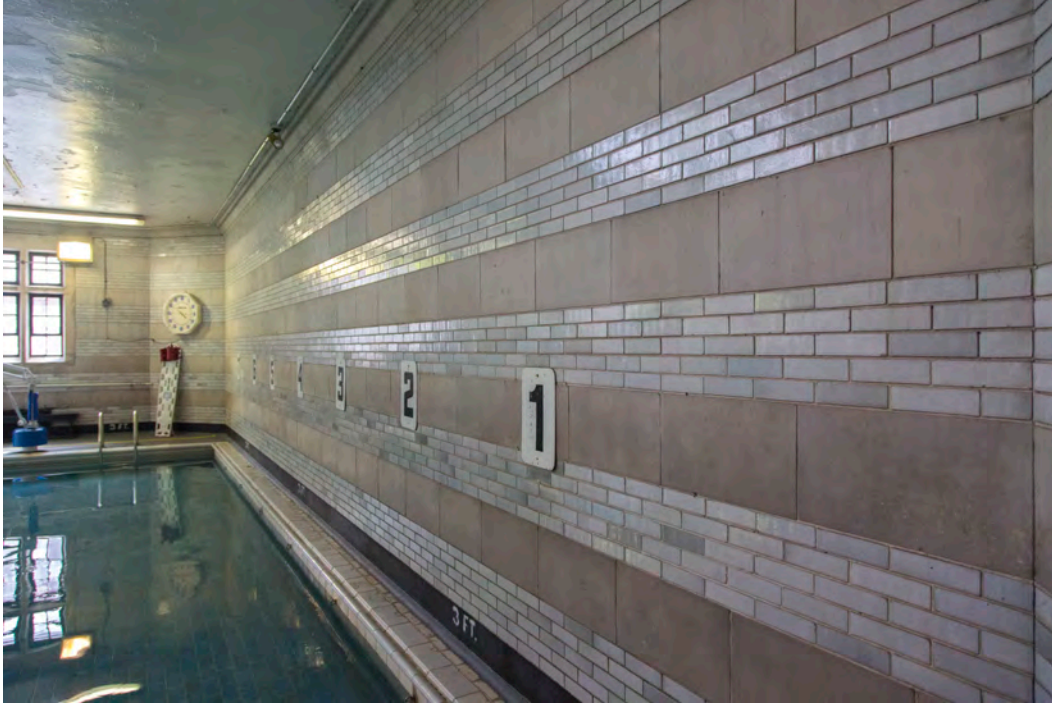
Photograph 17. First Floor Wall Detail.
