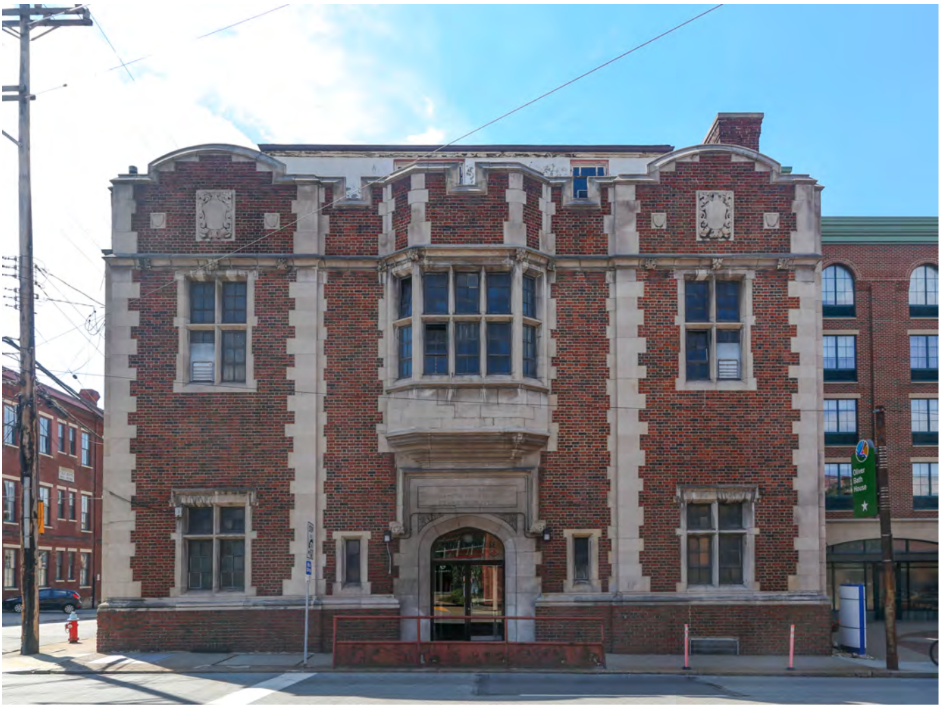
Photograph 1. Front (South 10th Street) Facade
