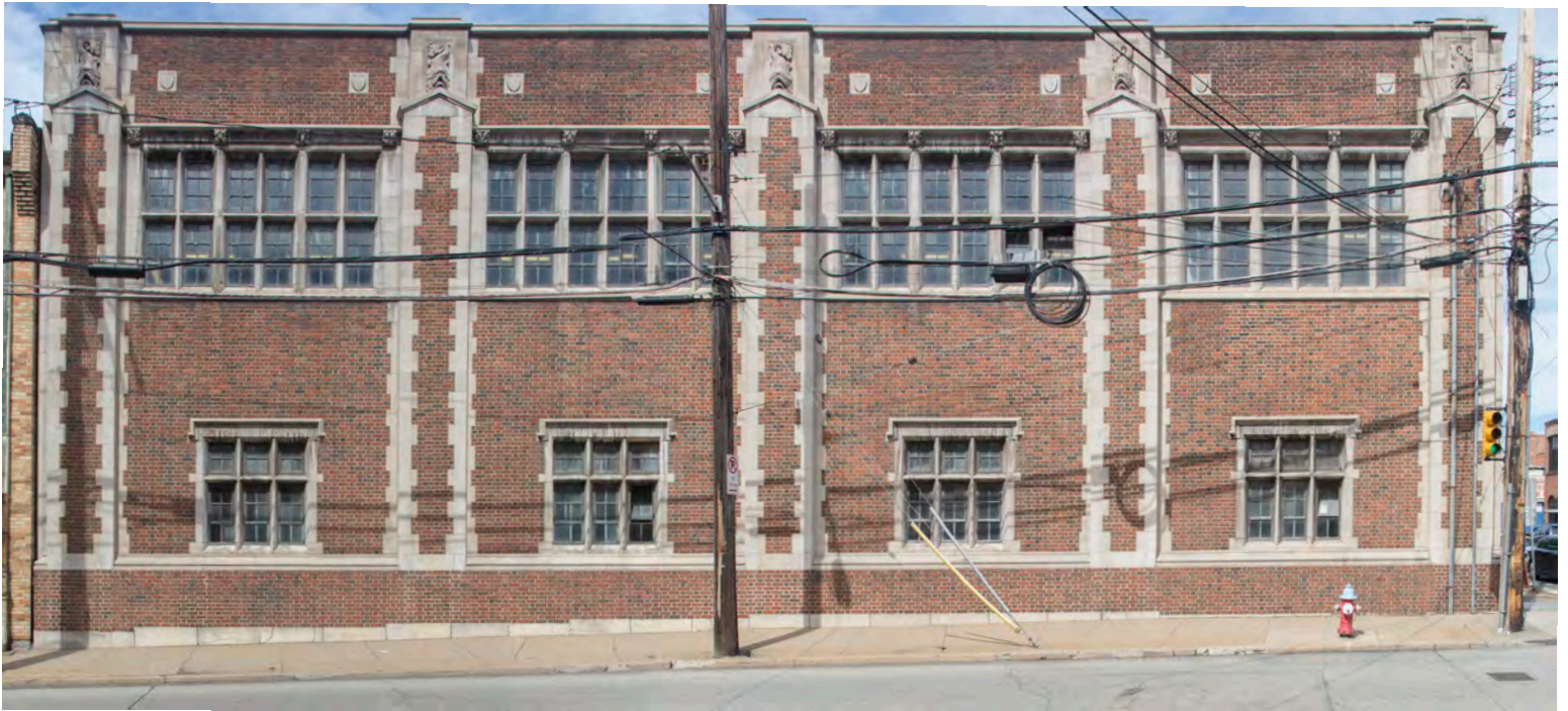
Photograph 2. Side (Bingham Street) Facade
