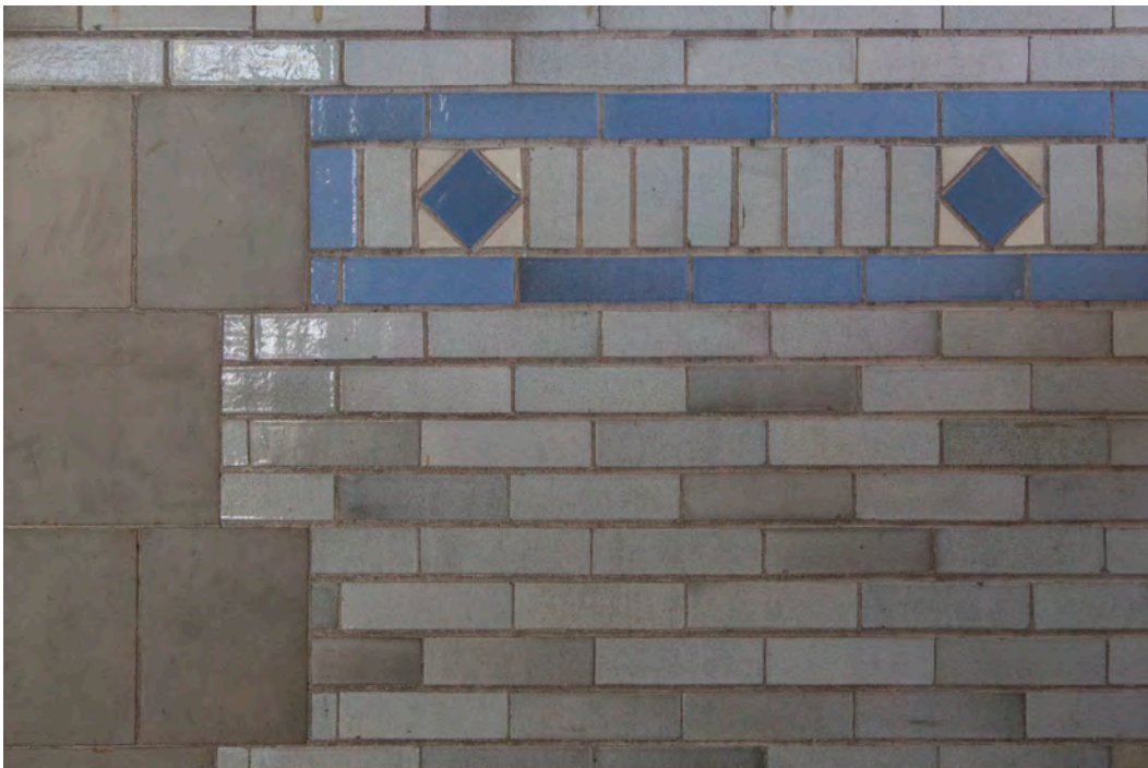
Photograph 18. Second Floor Wall Detail.
