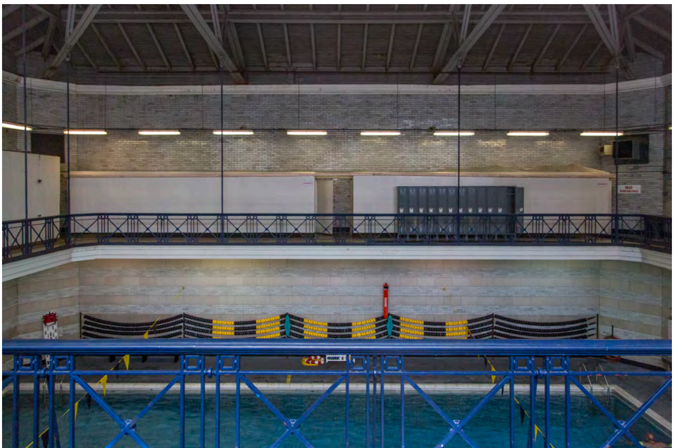
Photograph 6. Interior view from gallery level looking north.
