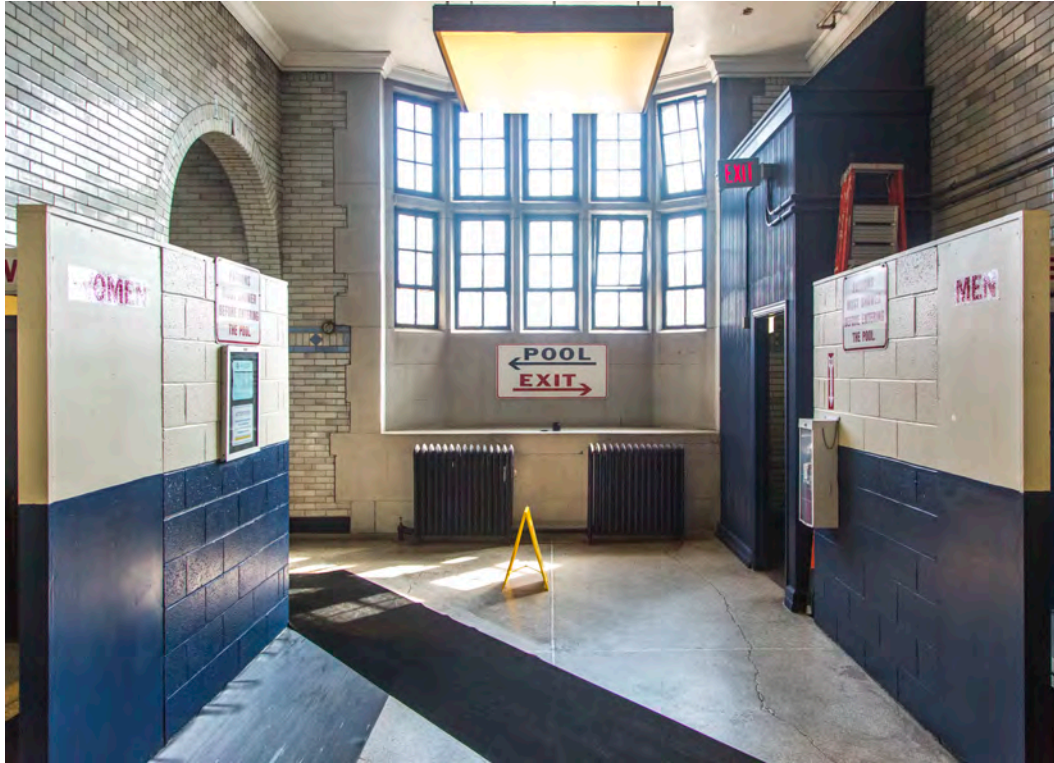
Photograph 9. Second Floor privacy walls outside toilets.
