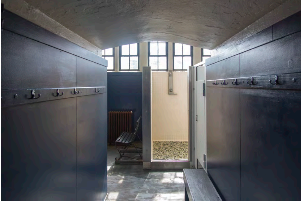
Photograph 13. Second Floor Men's Toilet.
