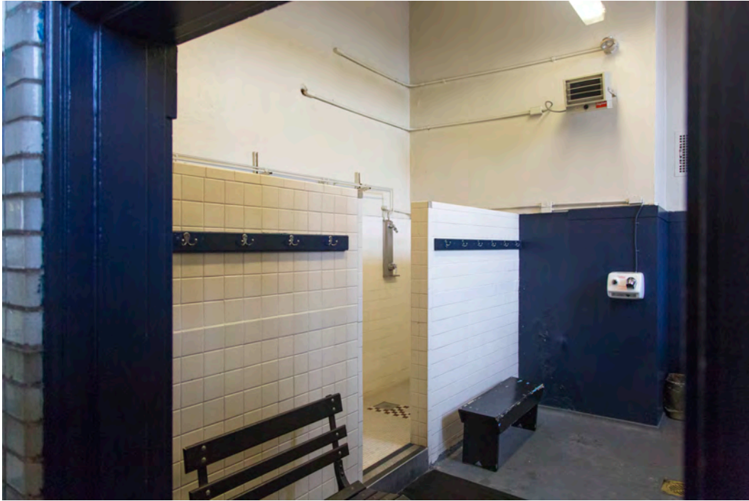
Photograph 11. View of Second Floor showers in Women's Toilet.
