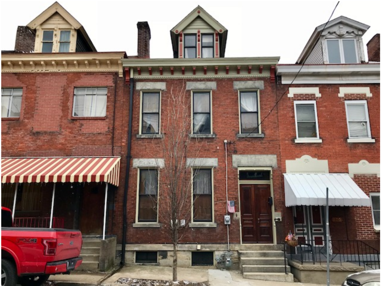
Photo. 2. Peterson House (172 46 th St.), Primary Façade, March 15, 2018. Source: Matthew W.C. Falcone.
