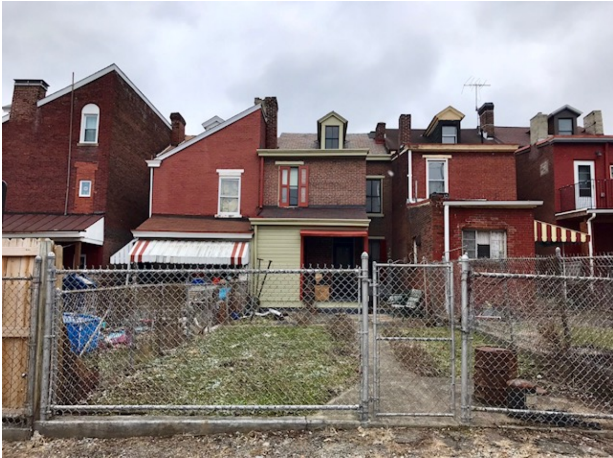
Photo. 6. Peterson House (172 46 th St.), Secondary Façade from Cotton Way, March 15, 2018. Source: Matthew W.C. Falcone.
