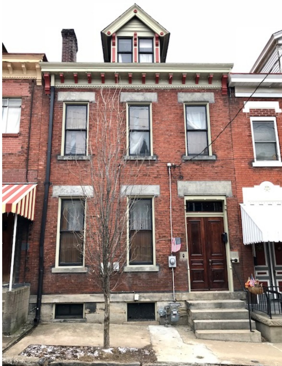
Photo. 1. Peterson House (172 46 th St.), Primary Façade, March 15, 2018. Source: Matthew W.C. Falcone.
