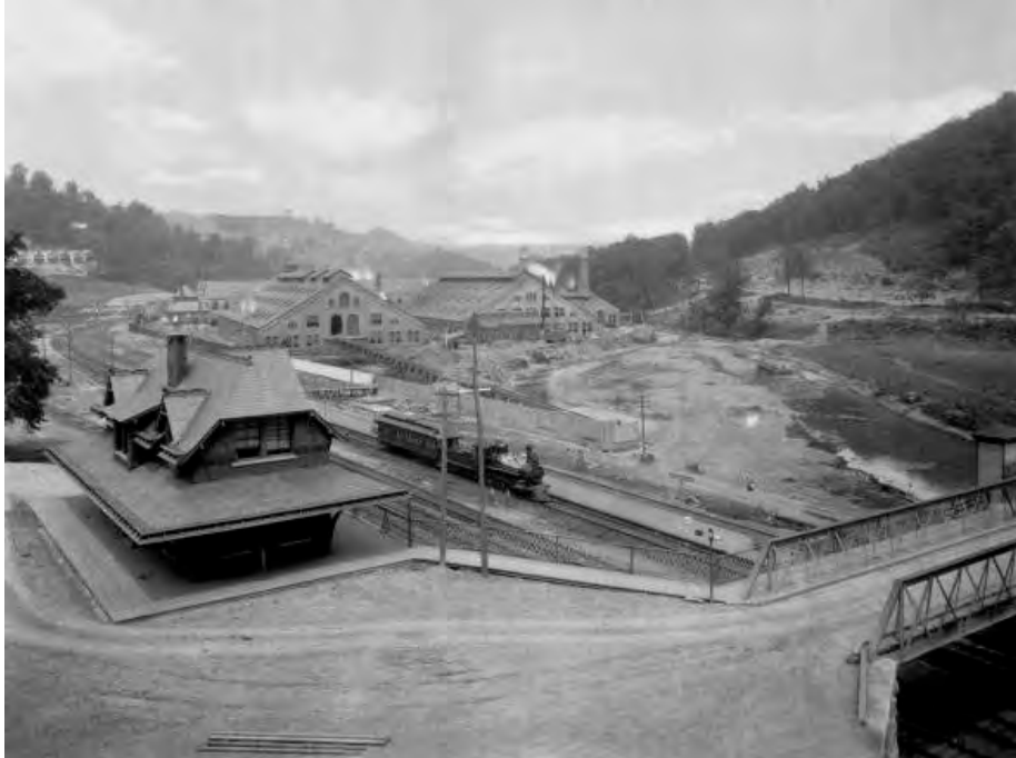
Fig. 10. Wilmerding Passenger Station , Source: http://www.west2k.com/papix/eastlibertypr.jpg (accessed on September 14, 2016).
