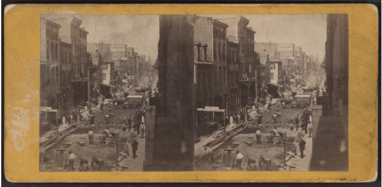
Fig. 28. Laying the Nicolson pavement in Mercer St., New York, E& H.T. Anthony, Source: https://en.wikipedia.org/wiki/Nicolson_pavement#/media/File:Laying_the_Nicolson_pavement_in_Mercer_St,_New_York,_by_E._%26_H.T._Anthony_%28Firm%29.jpg (accessed on September 14, 2016).
