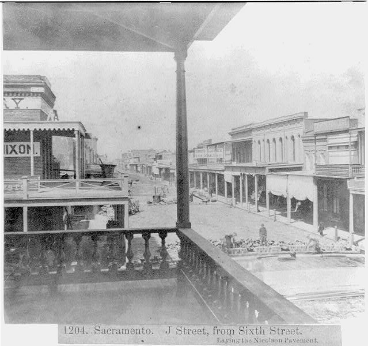
Figure 36: Sacramento, J Street from Sixth Street, Laying of the Nicolson Pavement.
