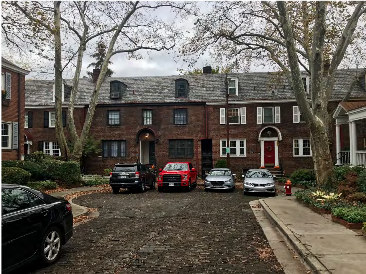
Figure 9: Roslyn Place (Taken from East Side of Cul-de-Sac, Facing West), November 1, 2019. Source: Matthew W.C. Falcone.
