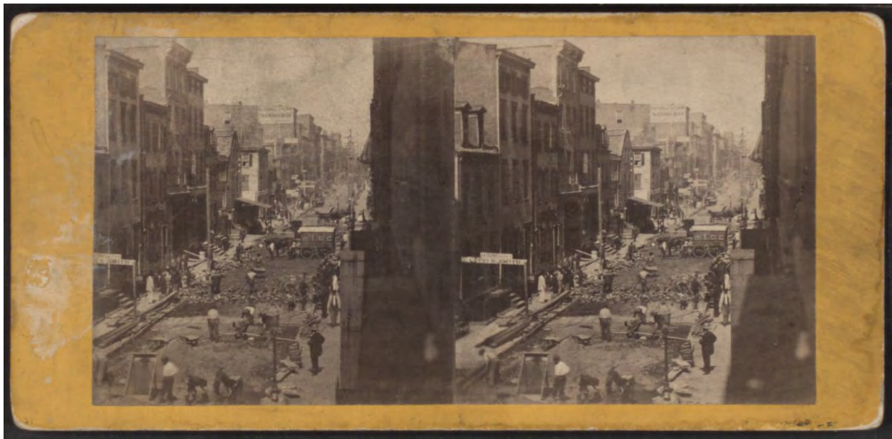
Figure 38: Laying the Nicolson pavement in Mercer St., New York, E& H.T. Anthony.
