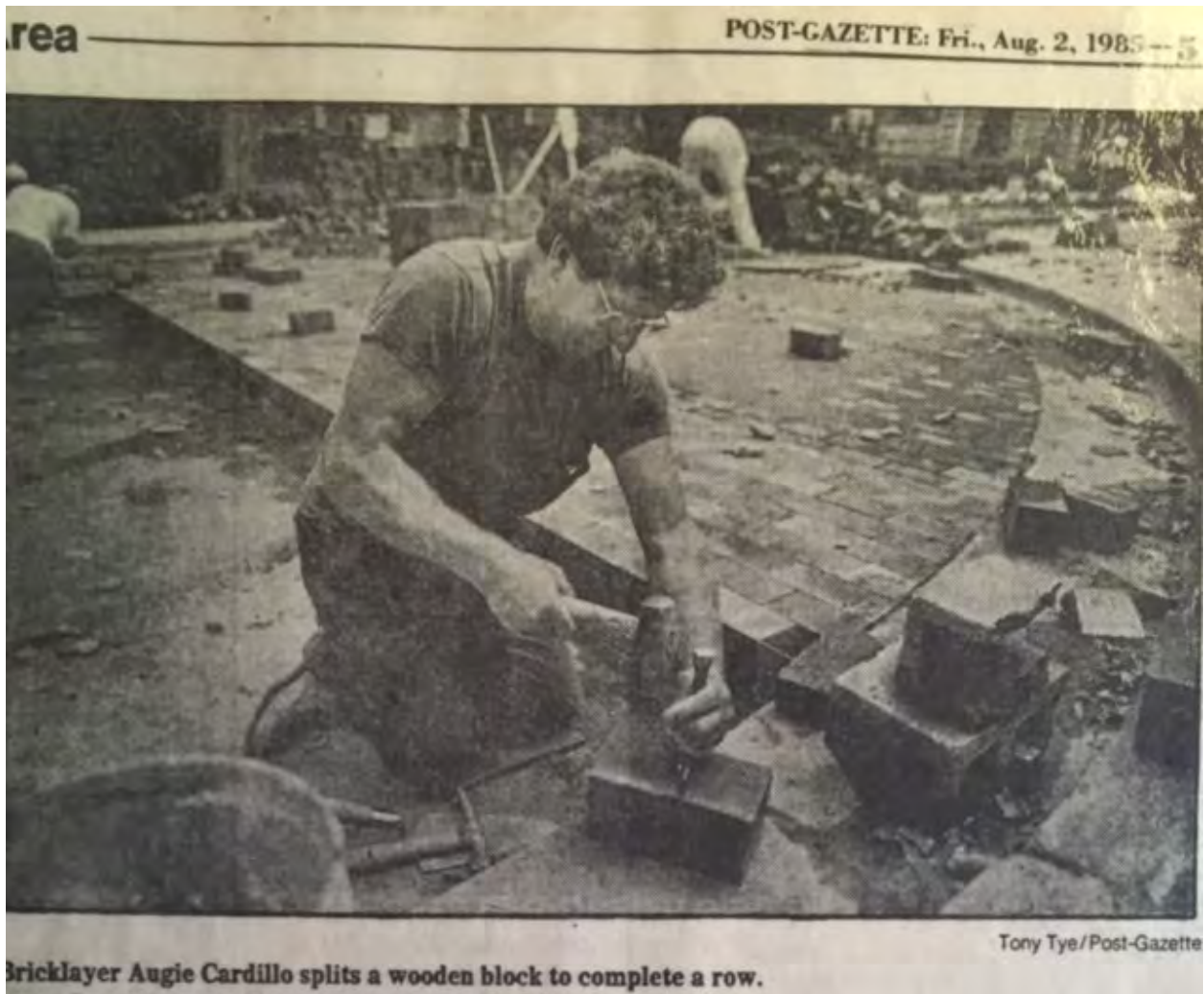
Figure 39: Bricklayer Augie Cardillo Splits a Wooden Block to Complete a Row, Pittsburgh Post-Gazette, August 2, 1985, from the private collection of Charlotte Cohen.
