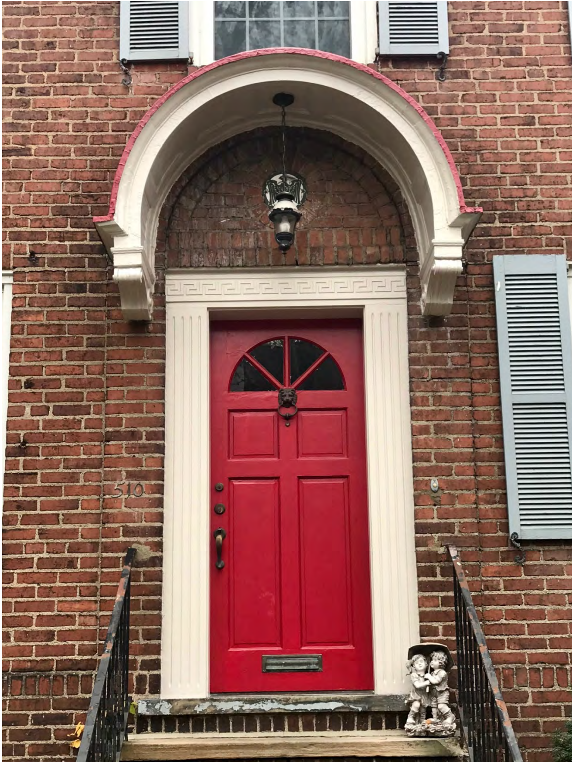
Figure 5: Door and Door hood, 512 Roslyn Place, November 1, 2019, Matthew W.C. Falcone.
