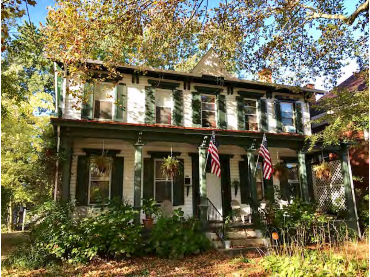
Photo. 1. 2803 Bergman St., Primary Façade, October 4, 2017. Source: Matthew W.C. Falcone.
