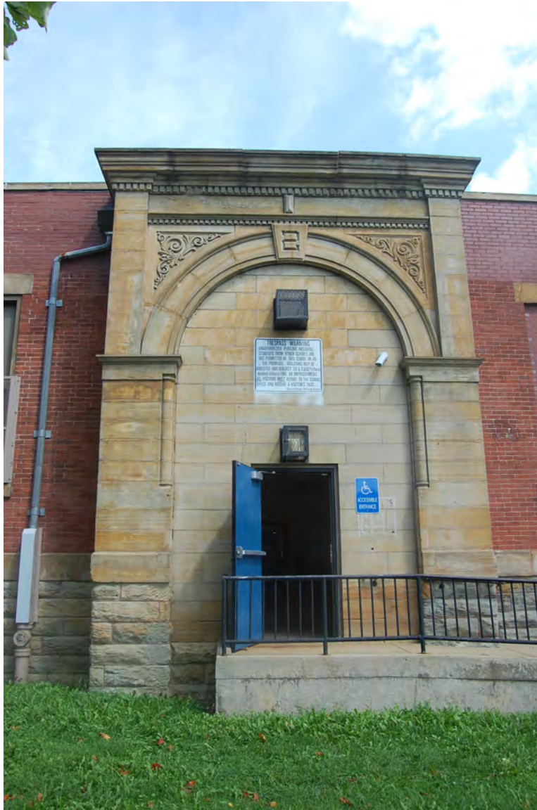
Photo 7. Original (ca. 1895) main entrance,
