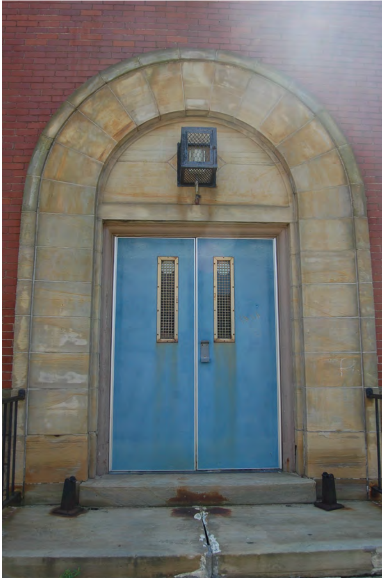
Photo 9. North facade entrance, west wing
