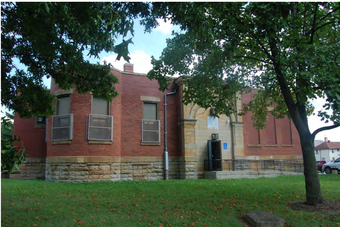
Photo 2. Original (1896) wing, west facade; first story and main entrance of original Spring Hill School building
