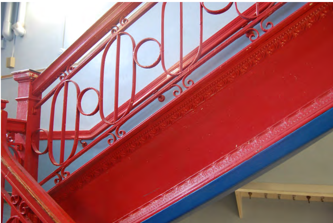
Photo 12. Staircase detail, east wing
