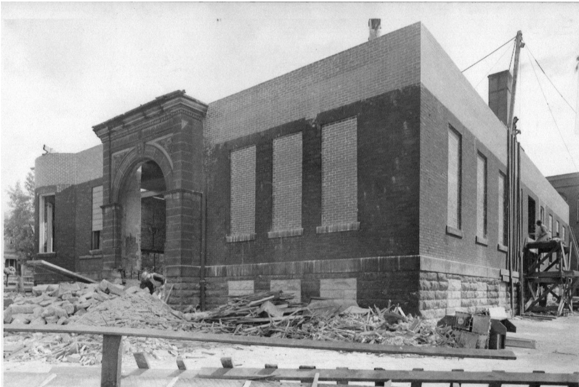
Fig. 9. Spring Hill School renovations in progress, 1936 (Pittsburgh Public Schools)
