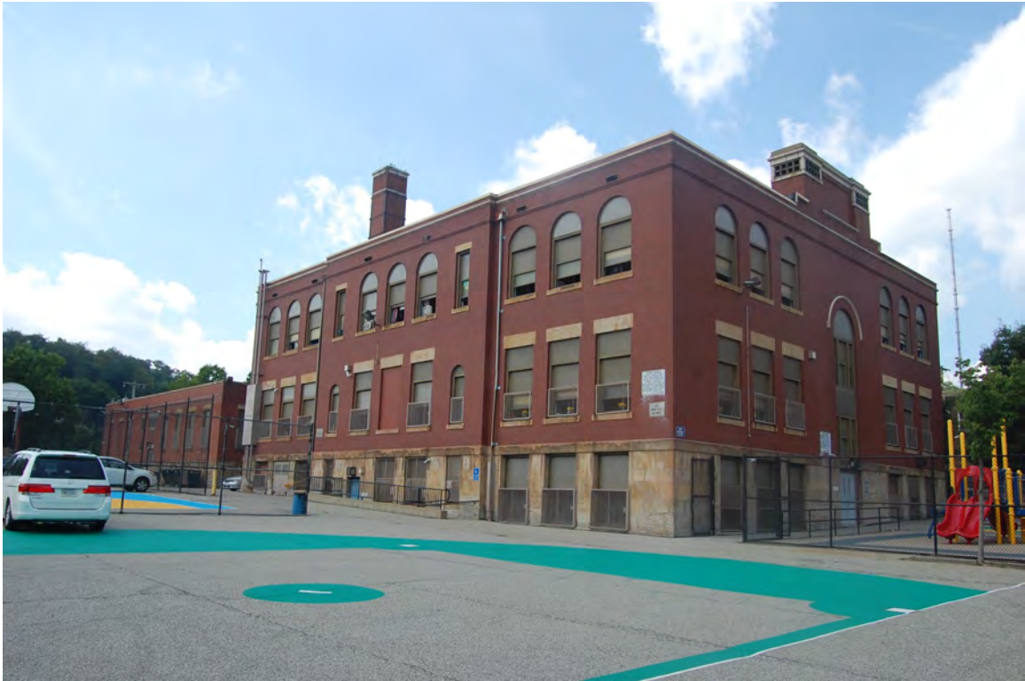
Photo 5. View of side and rear to northwest, 1908 building in foreground
