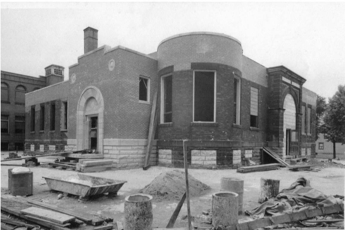
Fig. 10. Spring Hill School renovations in progress, 1936 (Pittsburgh Public Schools)
