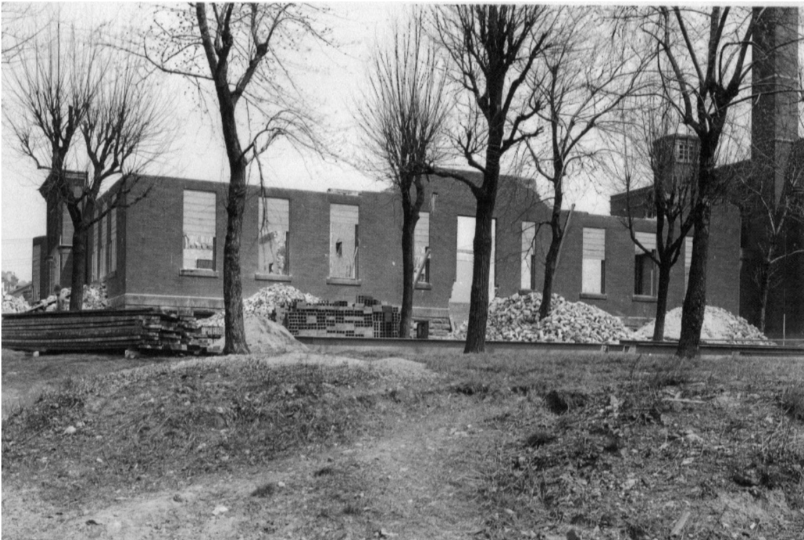
Fig. 7. Spring Hill School renovations in progress, 1936 (Pittsburgh Public Schools)
