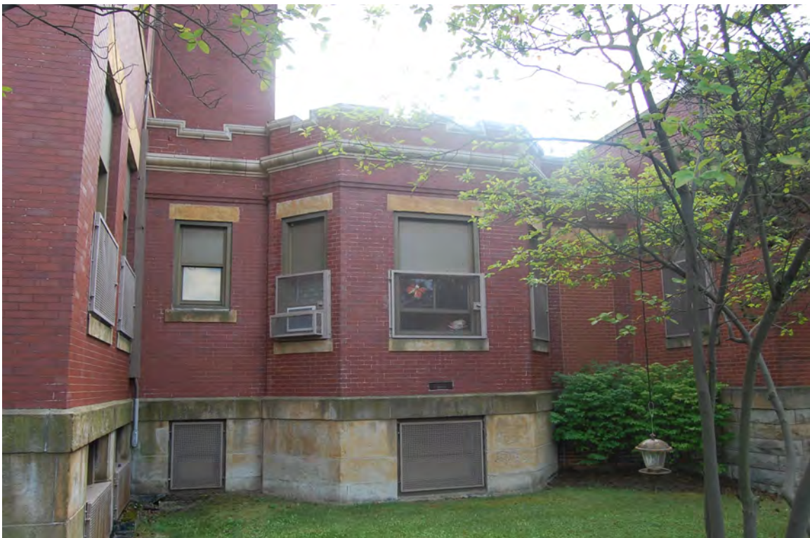
Photo 6. Connecting segment between 1896 and 1908 buildings, north facade
