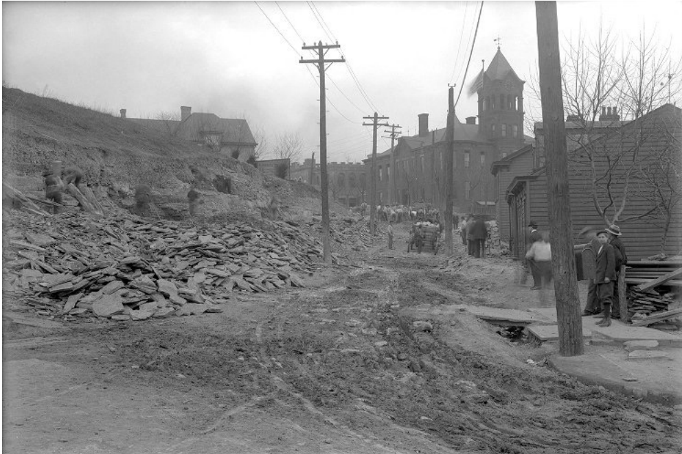
Fig. 5. Damas Street from Homer Street, looking east, 1912 Building at middle right with tower is original Spring Hill School 1908 addition with crenellated cornice visible beyond (Historic Pittsburgh)
