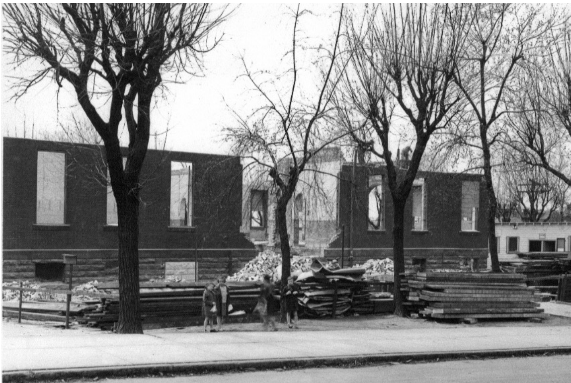
Fig. 8. Spring Hill School renovations in progress, 1936 (Pittsburgh Public Schools)
