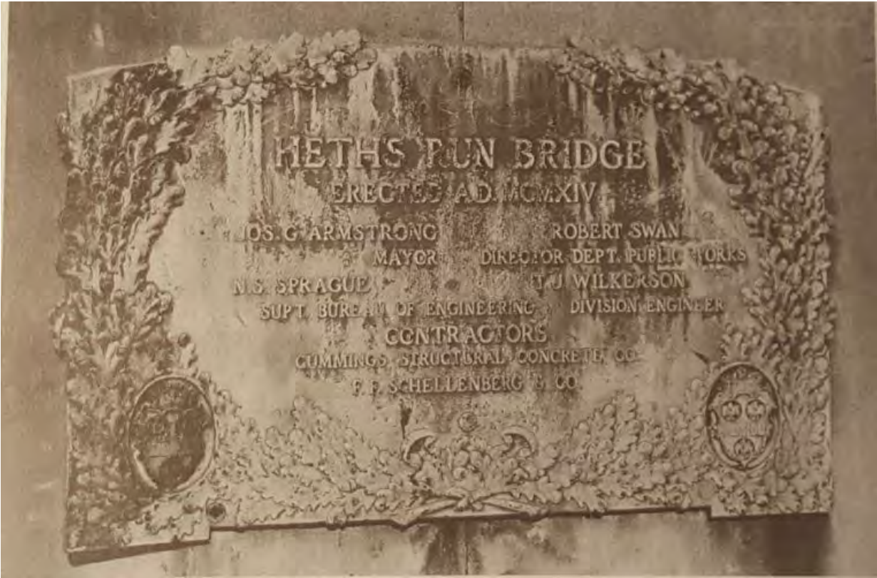
Fig. 17. Heth's Run Bridge Plaque, Source: Pittsburgh's Bridges: Architecture and Engineering
