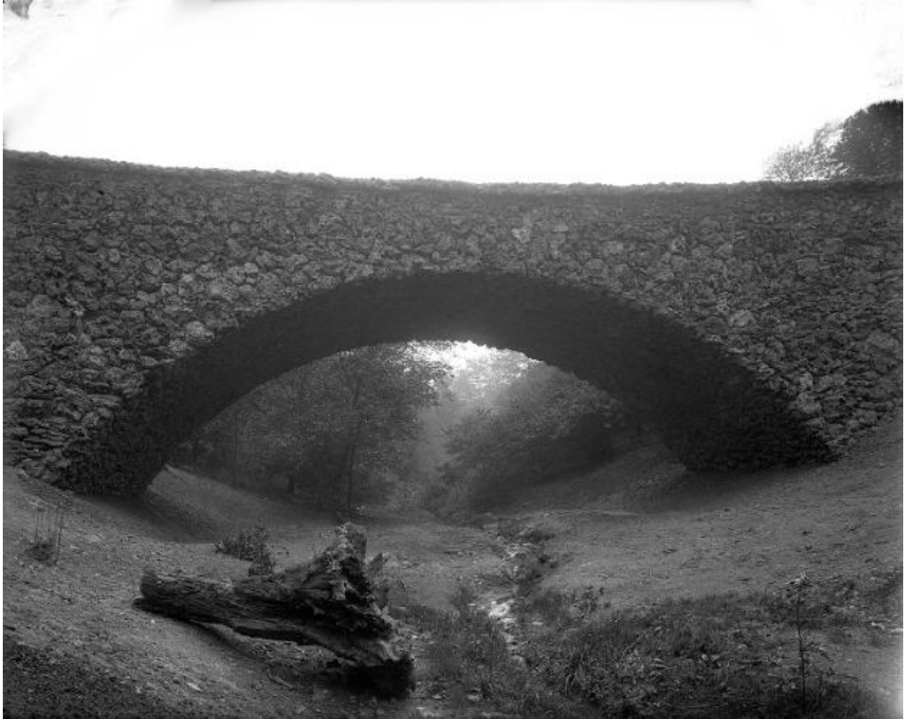
Fig. 5. Ravine – Rustic Bridge, September 14, 1908, Source: Pittsburgh City Photographer. http://histpitt.library.pitt.edu/islandora/object/pitt%3A715.087748.CP .
