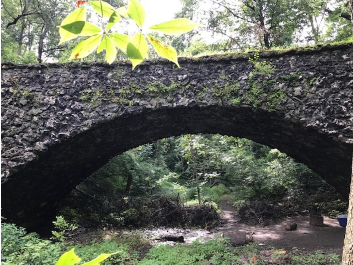
Photo. 1. Tufa Bridge II (Hemispherical Arch) , Schenley Park, June 2, 2017. Source: Matthew W.C. Falcone.
