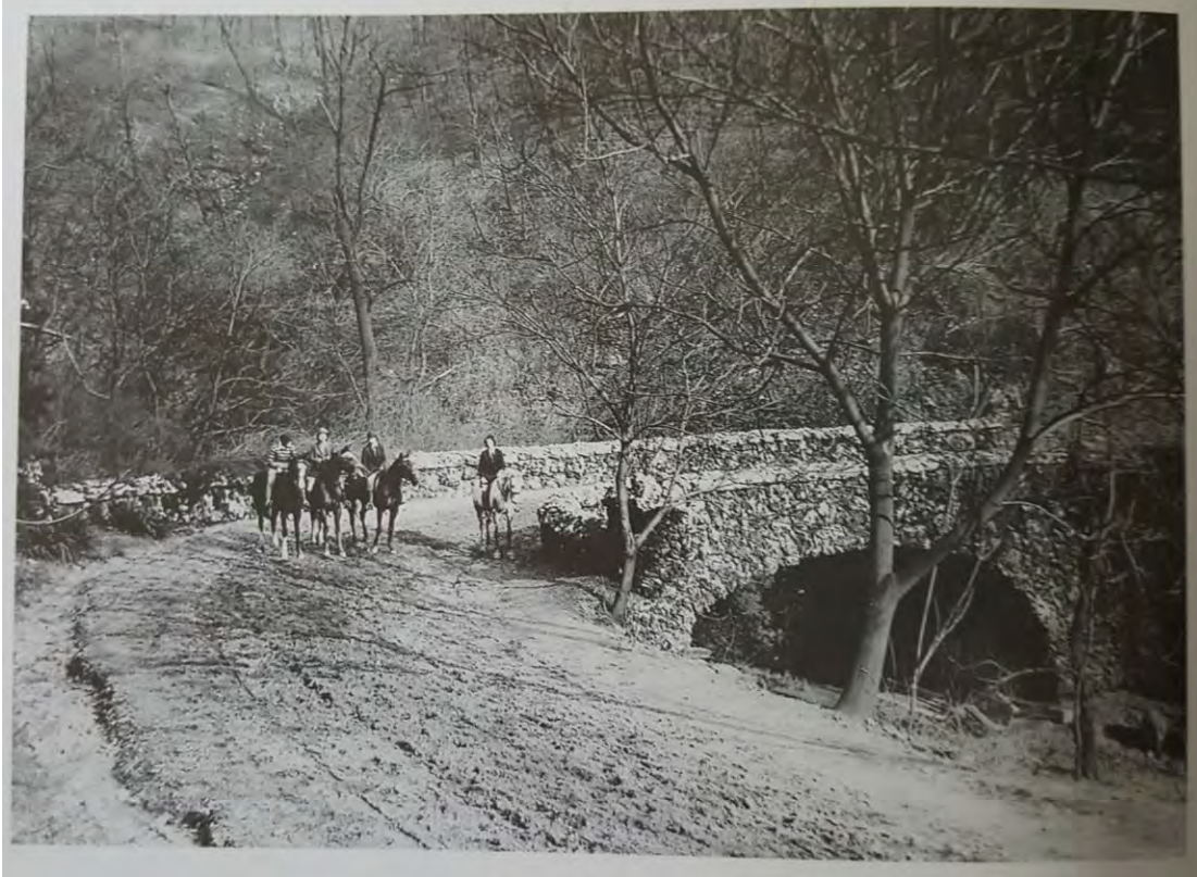
Fig. 44. Riding group at Upper Run Tufa Bridge, Source: Pittsburgh's Bridges: Architecture and Engineering by Walter Kidney
